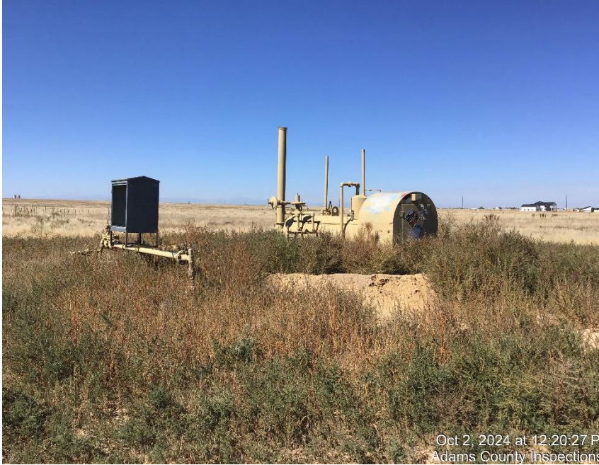
Photo #3 Meter run and separator (weeds throughout location).
