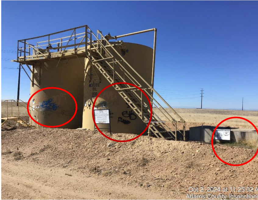
Photo #1 Tanks (weeds in and around berms and graffiti on tanks).
