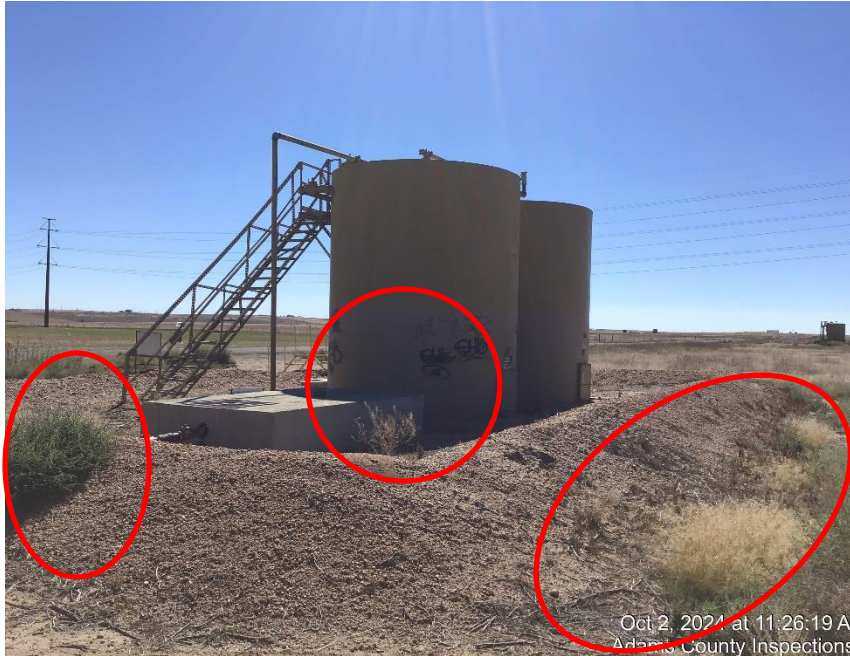
Photo #3 Tanks (weeds in and around berms and graffiti on tanks).
