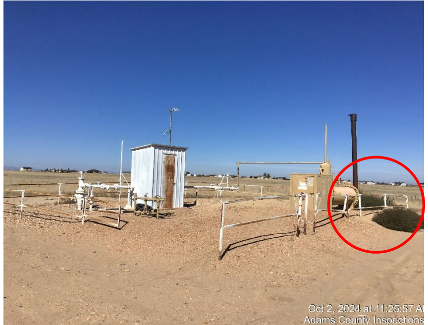
Photo #4 Meter house and separator (weeds around separator).
