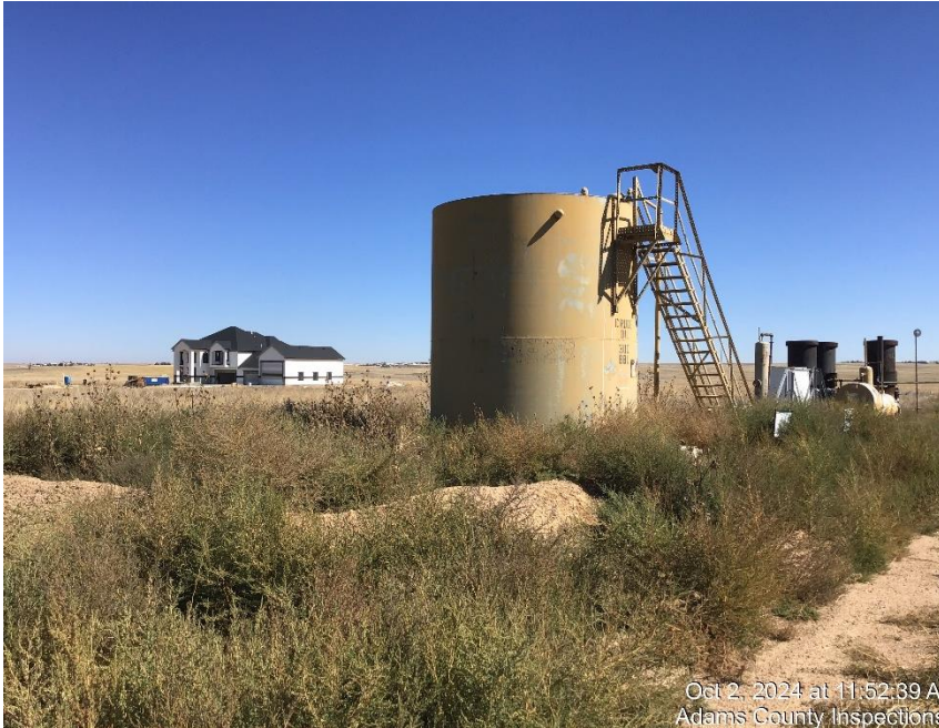
Photo #1 Tanks (weeds on, in and around berm, and throughout location).
