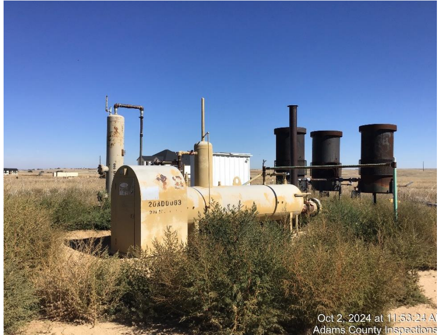
Photo #4 Separators, meter run and ECDs (weeds around equipment and throughout location).
