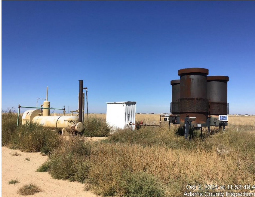
Photo #5 Separators, meter run and ECDs (weeds around equipment and throughout location).
