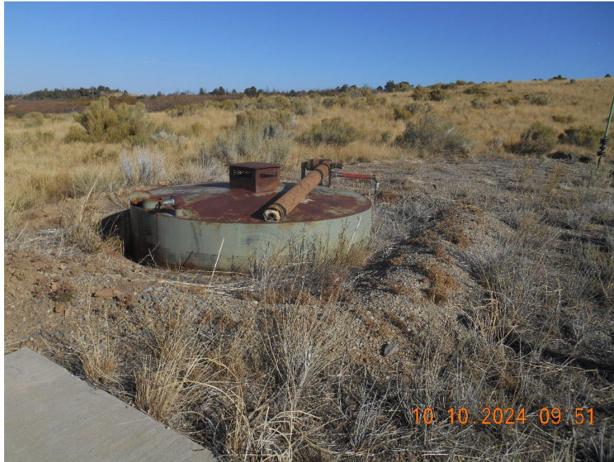
Blowdown tank for metering station
