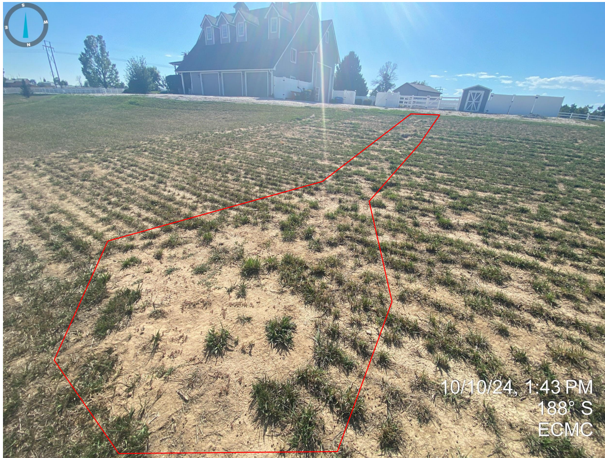
Photo 2. Photo taken from the eastern side of the disturbance area. Red polygon illustrates approximate extent of erosion degradation (e.g. riling) and sediment deposition in the reclaimed portions. Additional stormwater control measures and/or maintenance required to stabilize the soil and prevent sediment laden stormwater from exiting off location.
