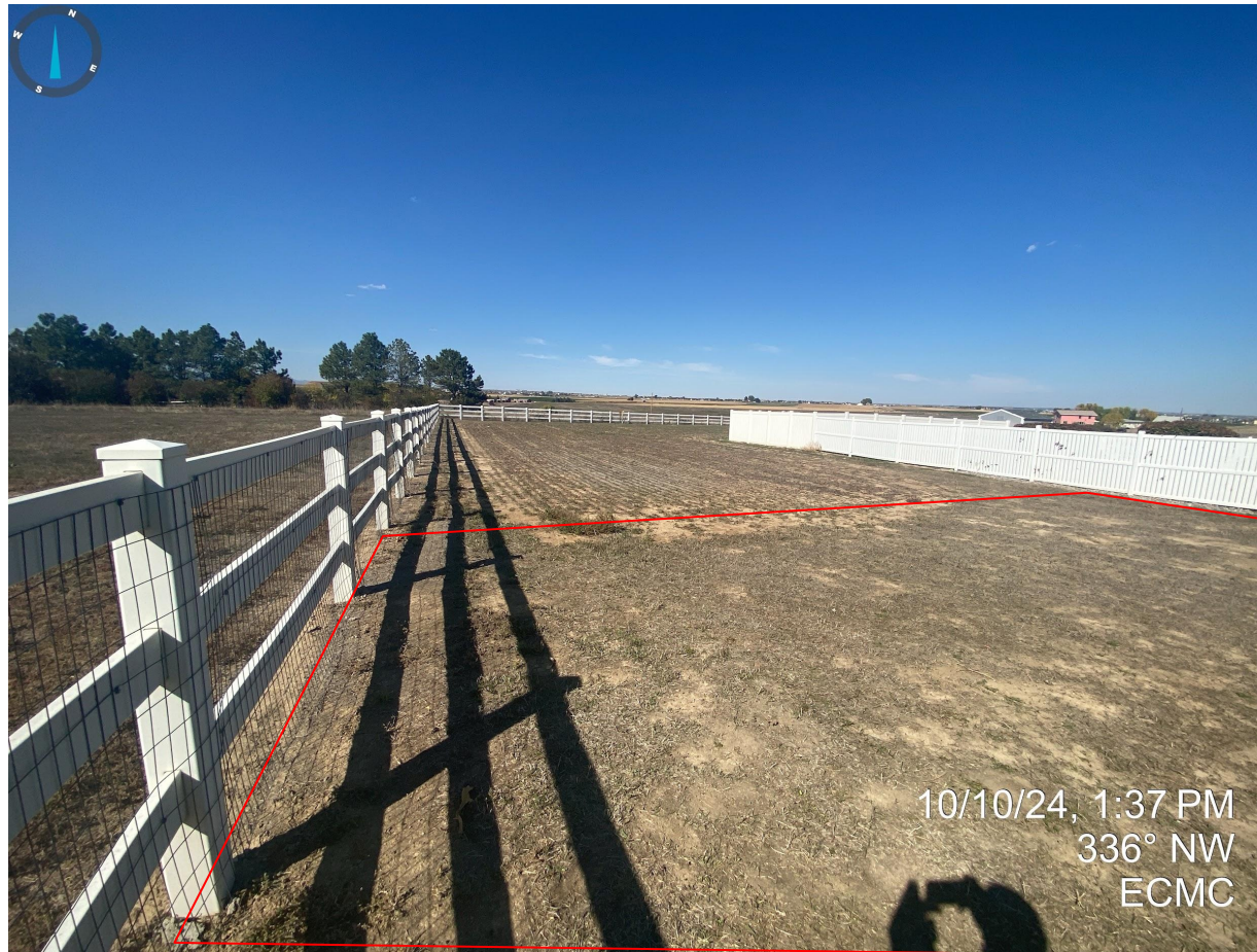
Photo 10. Southern/southwestern disturbance area. The outlined red polygon illustrates a portion of the disturbance area that does not appear to have been reclaimed; no evidence of drill rows and/or hydromulch observed.
