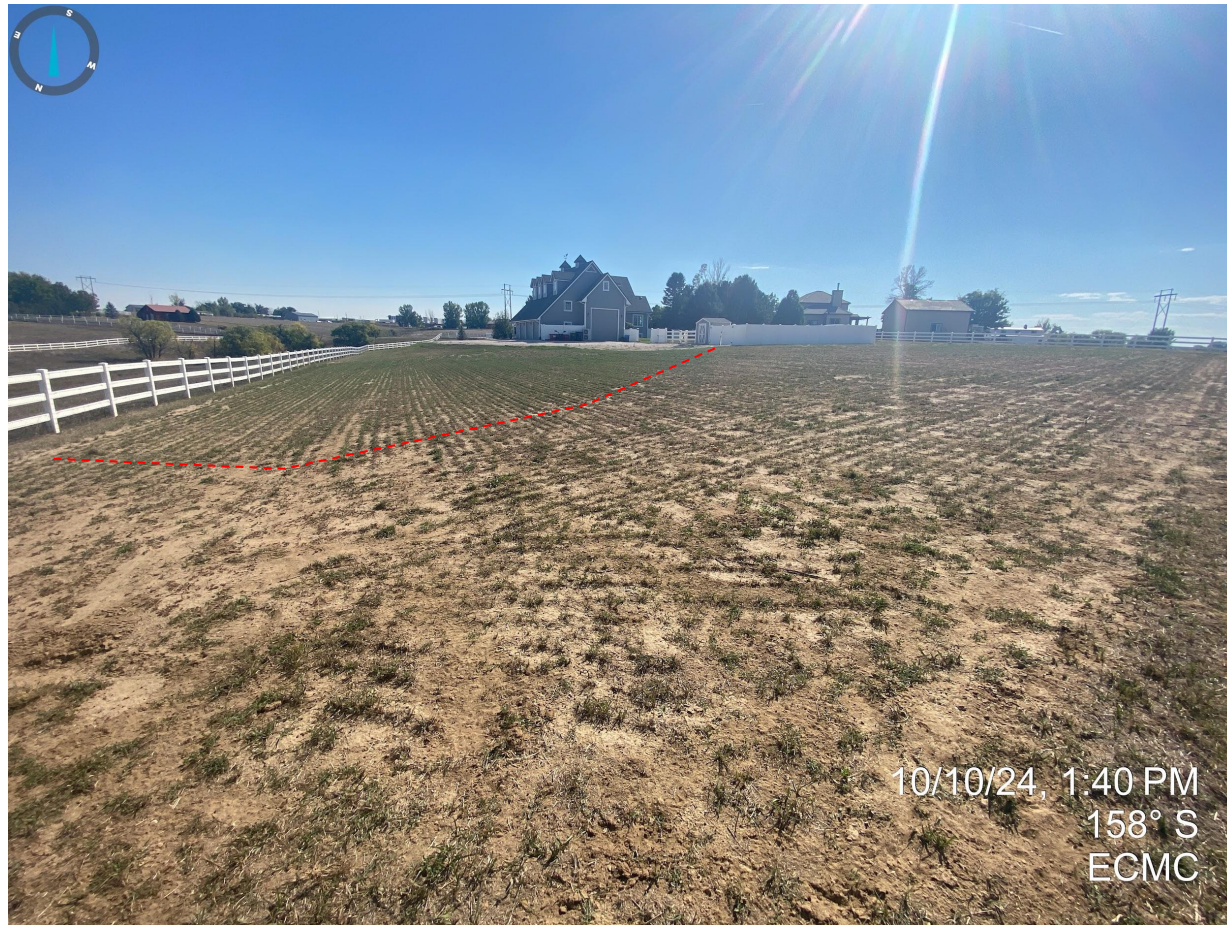
Photo 13. Northeastern disturbance areas; facing south. Photo illustrates the difference between the northern (right of dotted line) and eastern (left of dotted line) reclaimed portions. The northern areas do not appear to be progressing towards reclamation standards and regulations. Additional reclamation activities are required.
