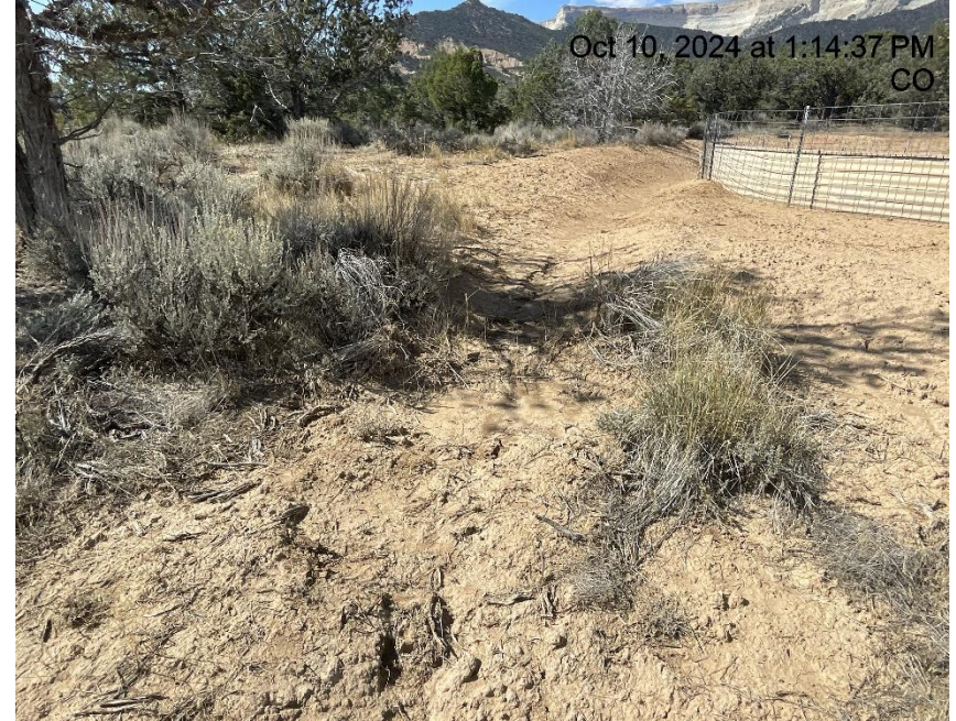
Photo # 4945 Failure to minimize erosion & transport of sediment off location - sediment laden stormwater is traveling through ditch & migrating off location into a vegetated area - insufficient BMP's/runoff controls.
