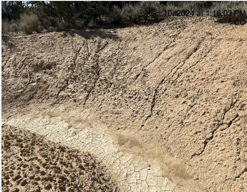
Photo # 4932 Erosion & transport of sediment on cut slope
