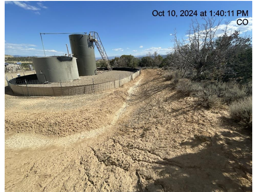
Photo # 4935 Erosion & transport of sediment on cut slope & insufficient BMP's/runoff controls
