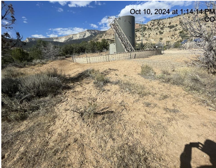
Photo # 4946 Failure to minimize erosion & transport of sediment off location - sediment laden stormwater is traveling through ditch & migrating off location into a vegetated area - insufficient BMP's/runoff controls.
