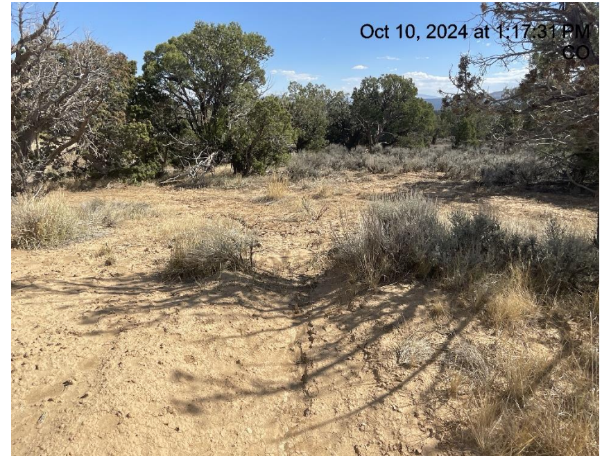
Photo # 4943 Failure to minimize erosion & transport of sediment off location - sediment laden stormwater is traveling through ditch & migrating off location into a vegetated area - insufficient BMP's/runoff controls.
