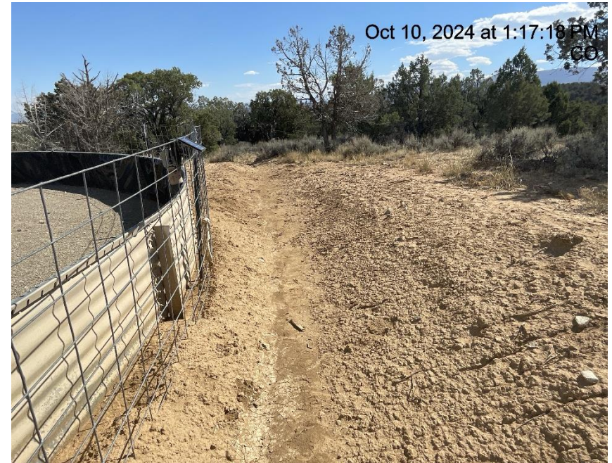
Photo # 4939 Failure to minimize erosion & transport of sediment off location - sediment laden stormwater is traveling through ditch & migrating off location into a vegetated area - insufficient BMP's/runoff controls.
