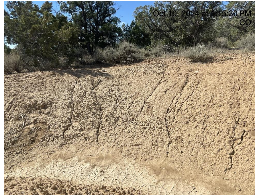
Photo # 4933 Erosion & transport of sediment on cut slope
