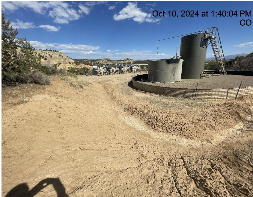
Photo # 4934 Erosion & transport of sediment on cut slope & insufficient BMP's/runoff controls
