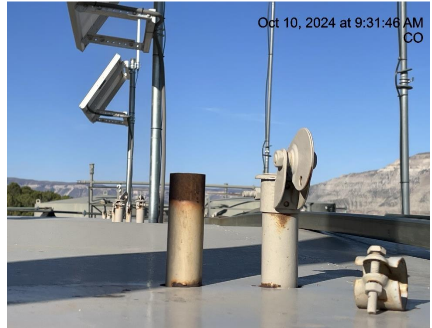
Photo # 4525 PRV vent line does not comply with CECMC pressure safety device rules
