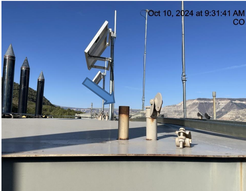
Photo # 4524 PRV vent line does not comply with CECMC pressure safety device rules
