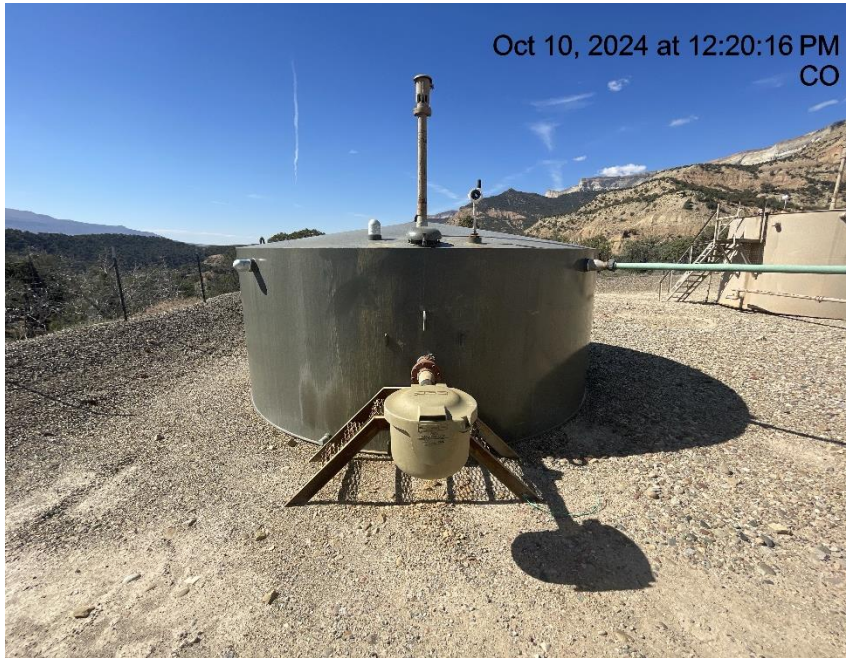
Photo # 4784 Production tank lacks required labeling
