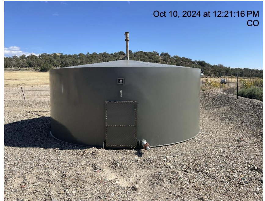
Photo # 4785 Production tank lacks required labeling
