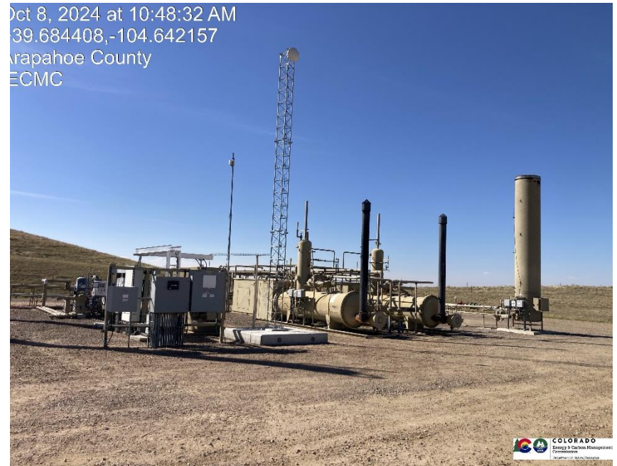
Pic 4 VRU, Separators, ECD, automation
