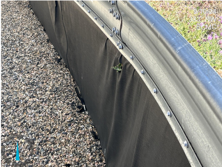
Photo 9. Photo taken from the southeast working pad at tank battery secondary containment. Photo illustrates that the liner is inadequate. Comply with Rule 603.o.
