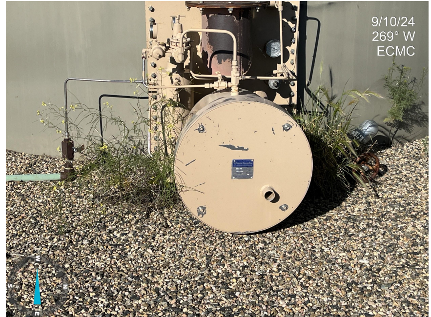
Photo 10. Photo taken from the tank battery. Photo illustrates missing caps/covers on equipment. Operator shall implement wildlife BMPs. Operator shall also manage weeds. Comply with Rule 902.b. and 606.
