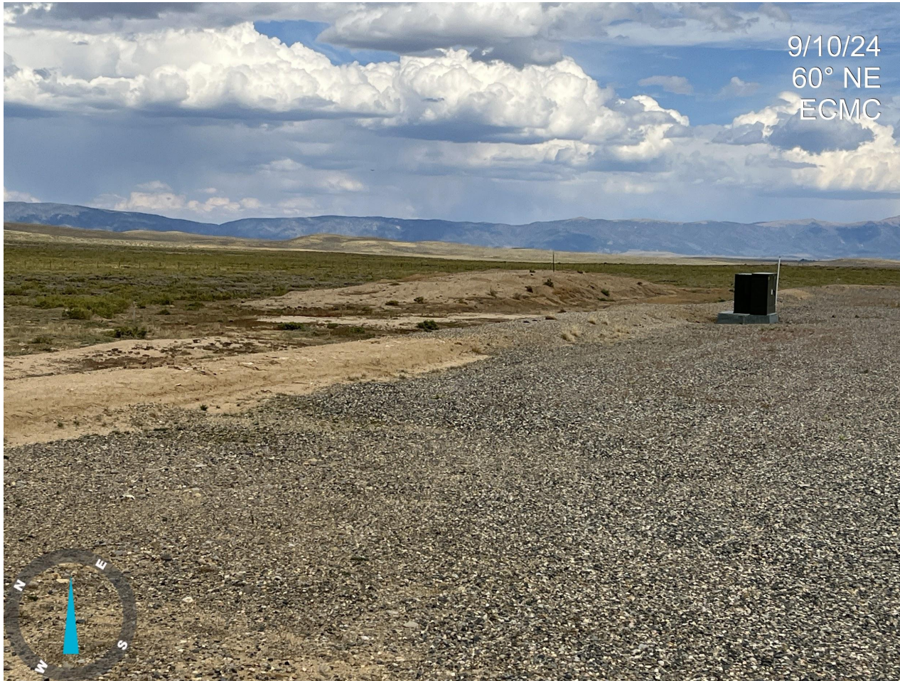
Photo 5. Photo taken from the western pad edge, facing NE. Photo illustrates insufficient or missing perimeter BMPs. Operator shall comply with Rules 1002.f.
