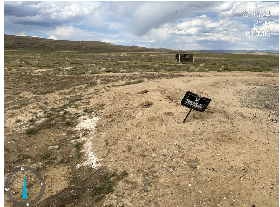
Photo 4. Photo taken from the western pad surface, facing north. Photo illustrates failing BMPs. Operator shall install/maintain stormwater BMPs per Rule 1002.f.
