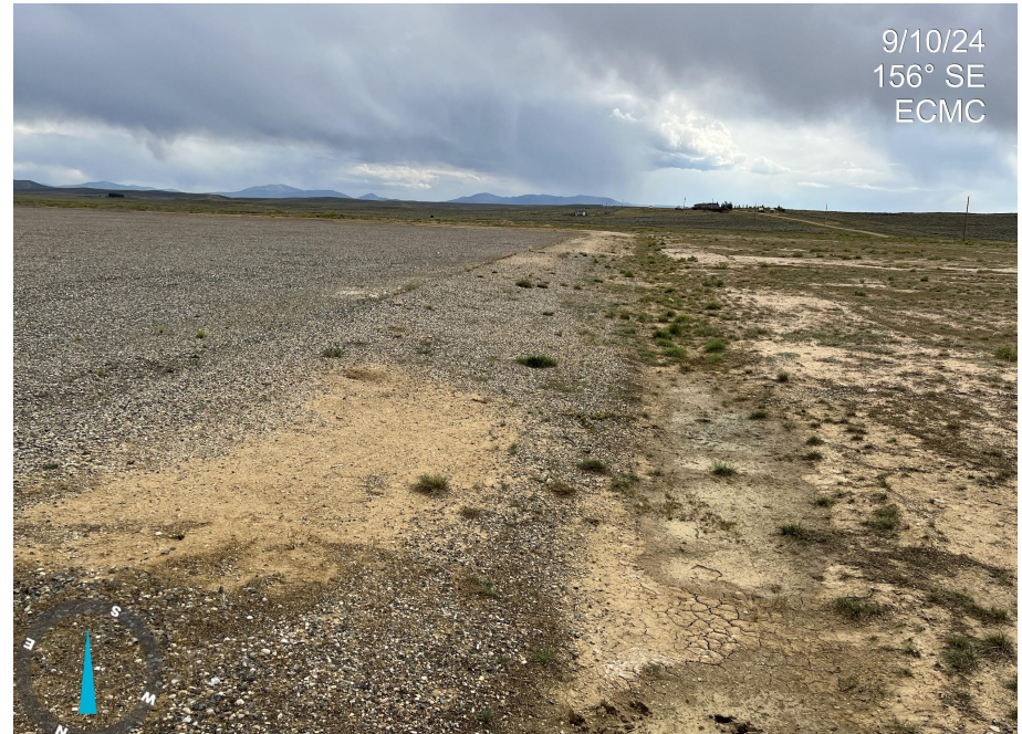
Photo 2. Photo taken the entrance of the Location, facing SE. Weeds observed growing along the perimeter. Photo illustrates failure of stormwater BMPs. Evidence of stormwater run-off outside of pad. Operator shall repair stormwater BMPs per Rule 1002.f.
