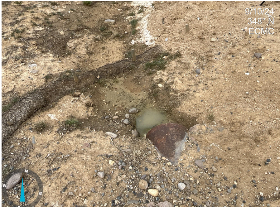
Photo 3. Photo taken from the western pad surface, facing north. Photo illustrates erosion. Operator shall install/maintain stormwater BMPs per Rule 1002.f.(2)
