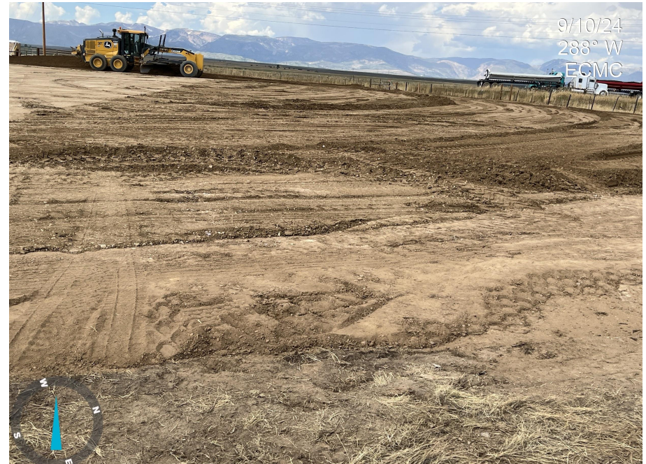
Photo 2. Photo taken from the eastern edge of Location facing west. Photo illustrates construction grading without perimeter stormwater BMPs
