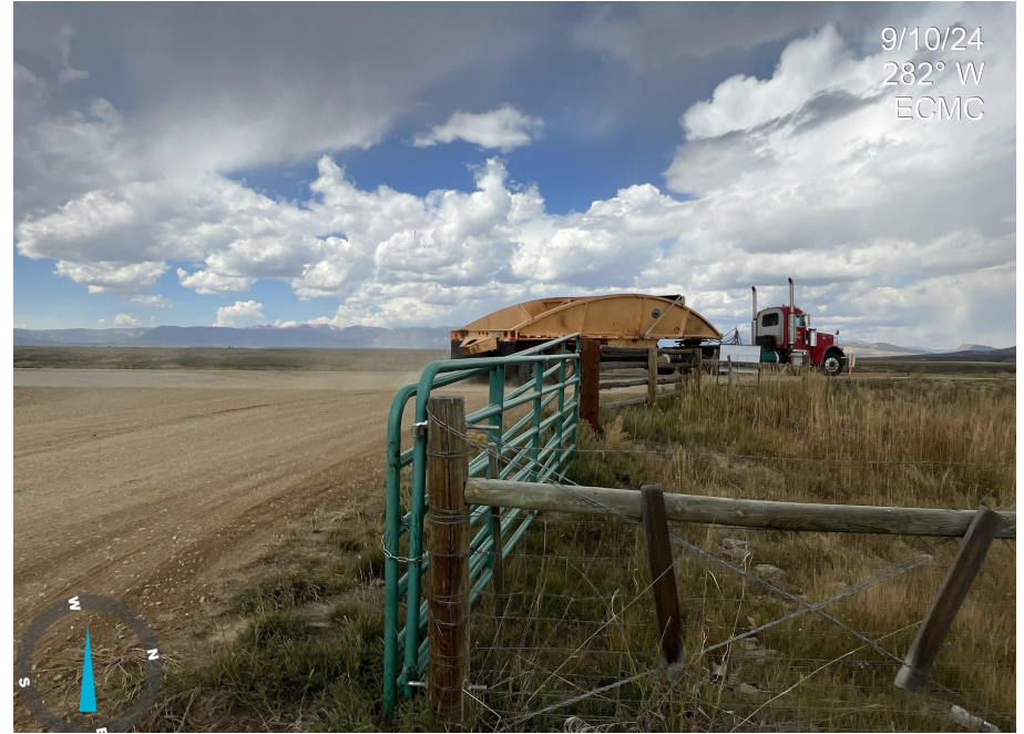
Photo 4. Photo taken from the entrance of Location facing Highway 14. Tracking pad not installed to prevent track of material off site. Discussion with Operator that street sweeper was employed to clean sediment tracked off-site.
