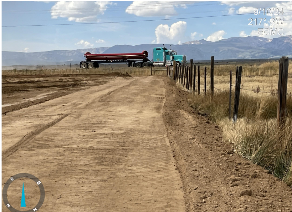
Photo 5. Photo taken from the northeastern edge of Location, facing southwest. Photo illustrates Location perimeter. No stormwater perimeter BMPs installed prior to construction, per Rule 1002.f.(2) .
