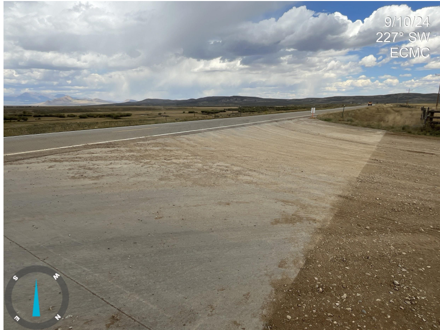
Photo 3. Photo taken from the entrance of Location facing Highway 14. Photo illustrates sediment track-out offsite. Sediment transport was not observed at longer distances away from entrance.
