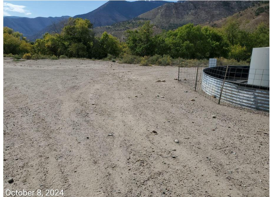
**Photo 1:** Operator appears to have performed grading operations to address tracking and stabilization concerns. Unclear if controls are adequate to address the tracking and stabilization concerns during wet conditions.
