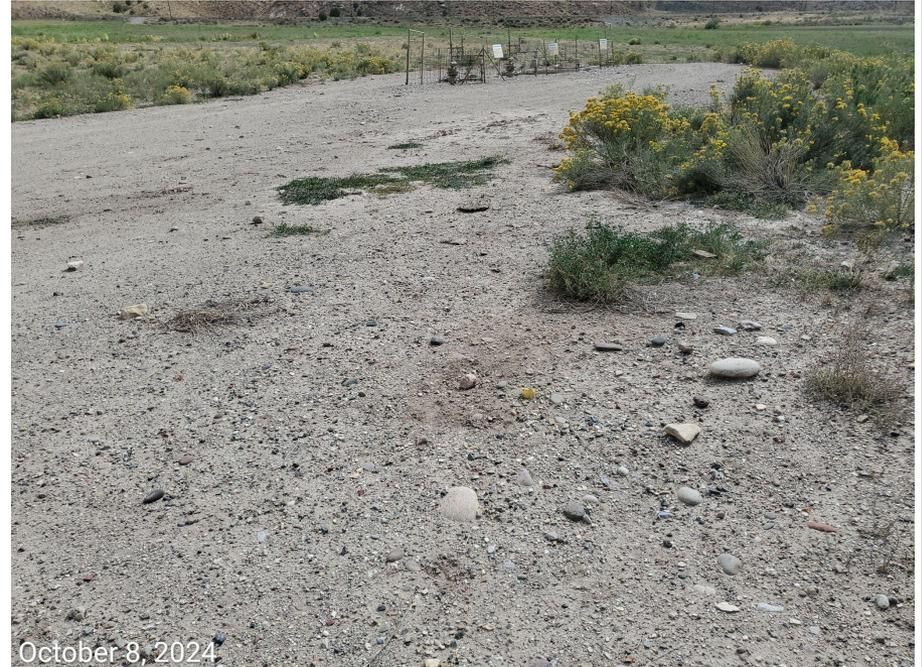
**Photo 3:** Anchor markers do not comport with 603.j/1003.a requirements.
