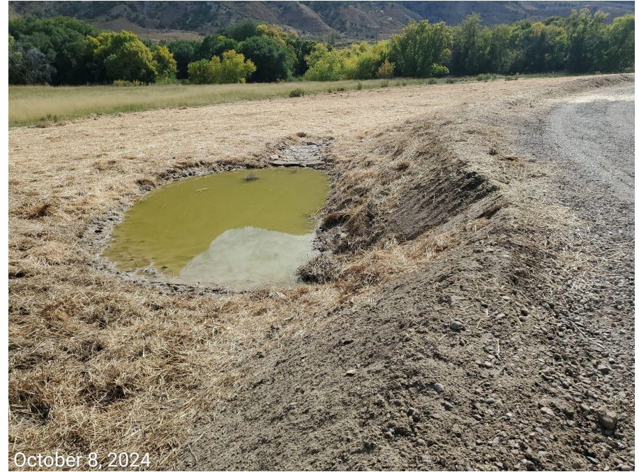
Photo 7: Examples of additional sediment traps implemented along the east end of the Location.
