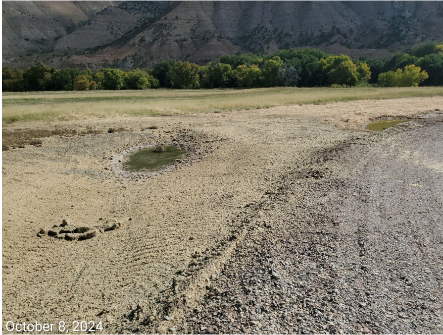
Photo 7: Examples of additional sediment traps implemented along the east end of the Location.
