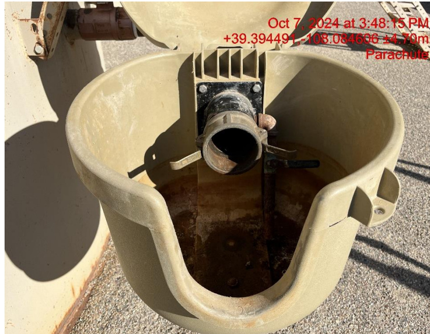
Photo # 7061 Open ended load line
