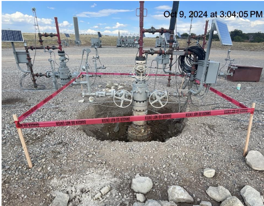
Photo # 4322 Insufficient wildlife protection for hole around wellhead/wildlife hazard
