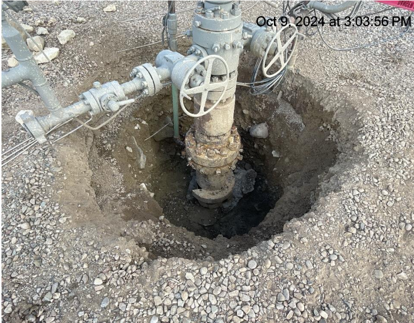
Photo # 4324 Insufficient wildlife protection for hole around wellhead/wildlife hazard
