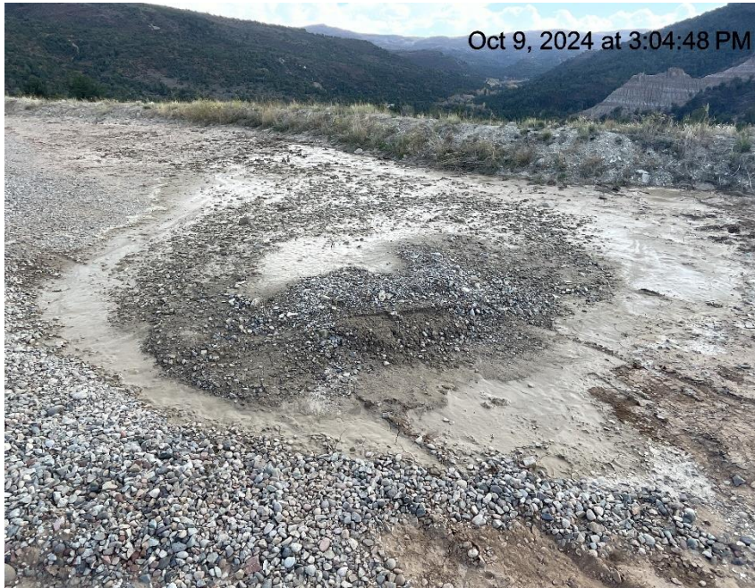
Photo # 4326 Stockpiled soils with no BMP's
