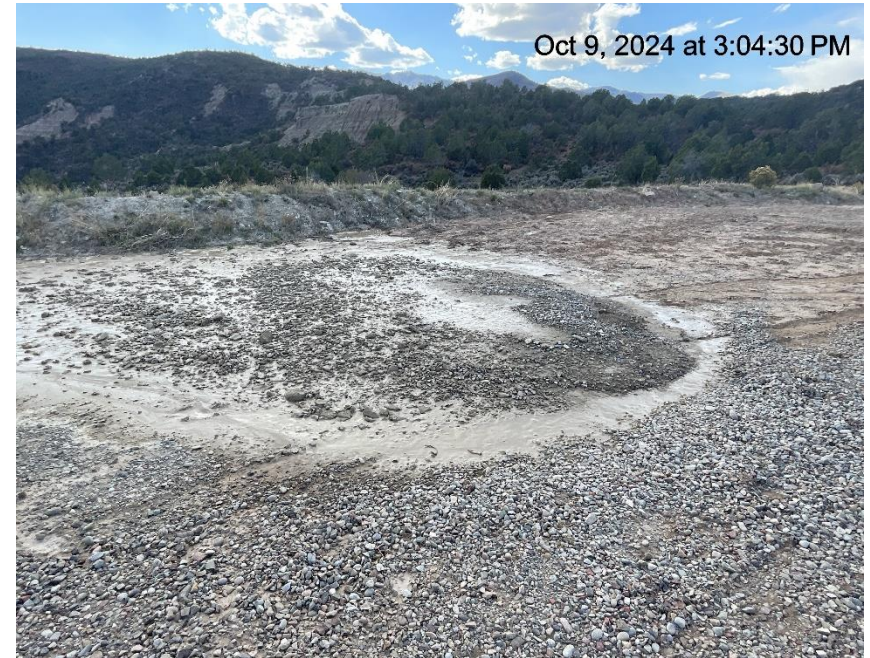
Photo # 4327 Stockpiled soils with no BMP's
