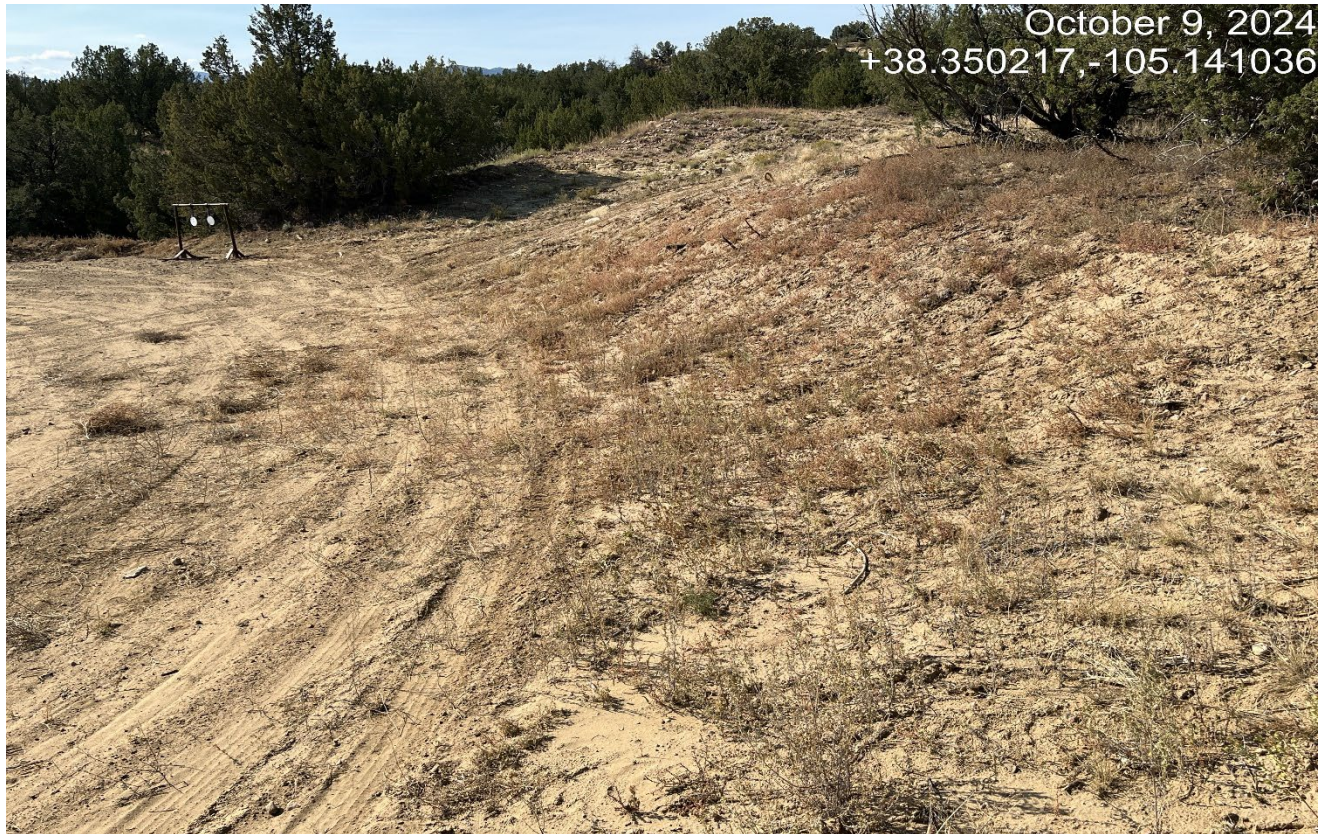
Photo 17. Facing southwest at the location. The cut slope of the location is not stabilized and there are insufficient stormwater run-on controls.
