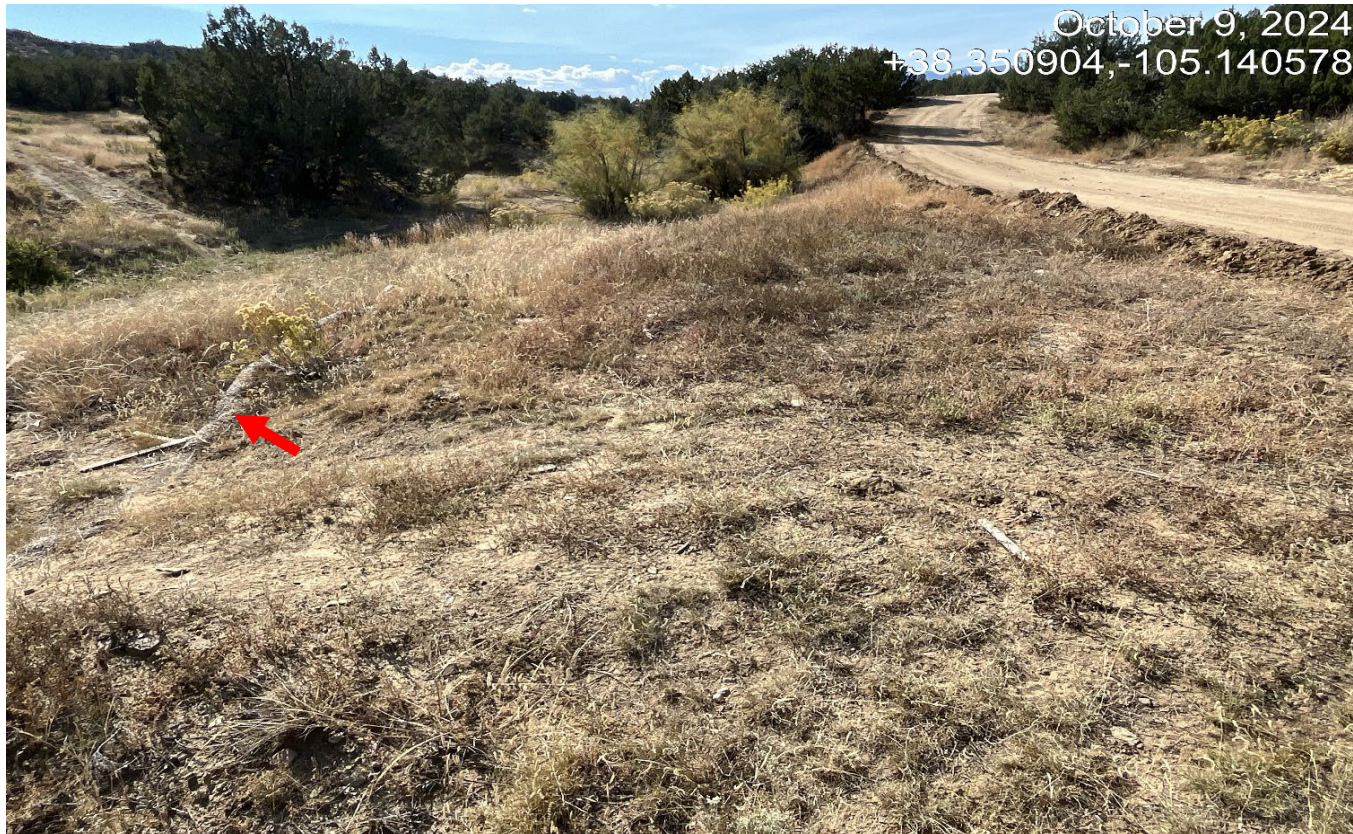
Photo 7. Facing south where soils were pushed out along the road side. This area needs to be reclaimed and perimeter wattles need maintenance shown at red arrow.
