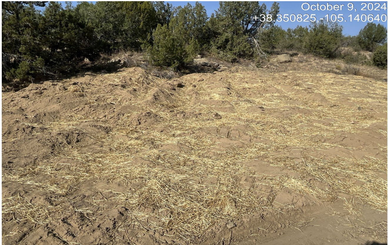
Photo 9. The soils were not leveled and remain loose and susceptible to erosion. The straw mulch is not crimped into the soils and can blow away.
