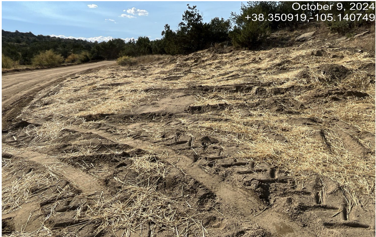
Photo 8. Facing south toward the tank battery site. The tanks have been removed and soils have been contoured. The soils were not leveled and remain loose and susceptible to erosion.
