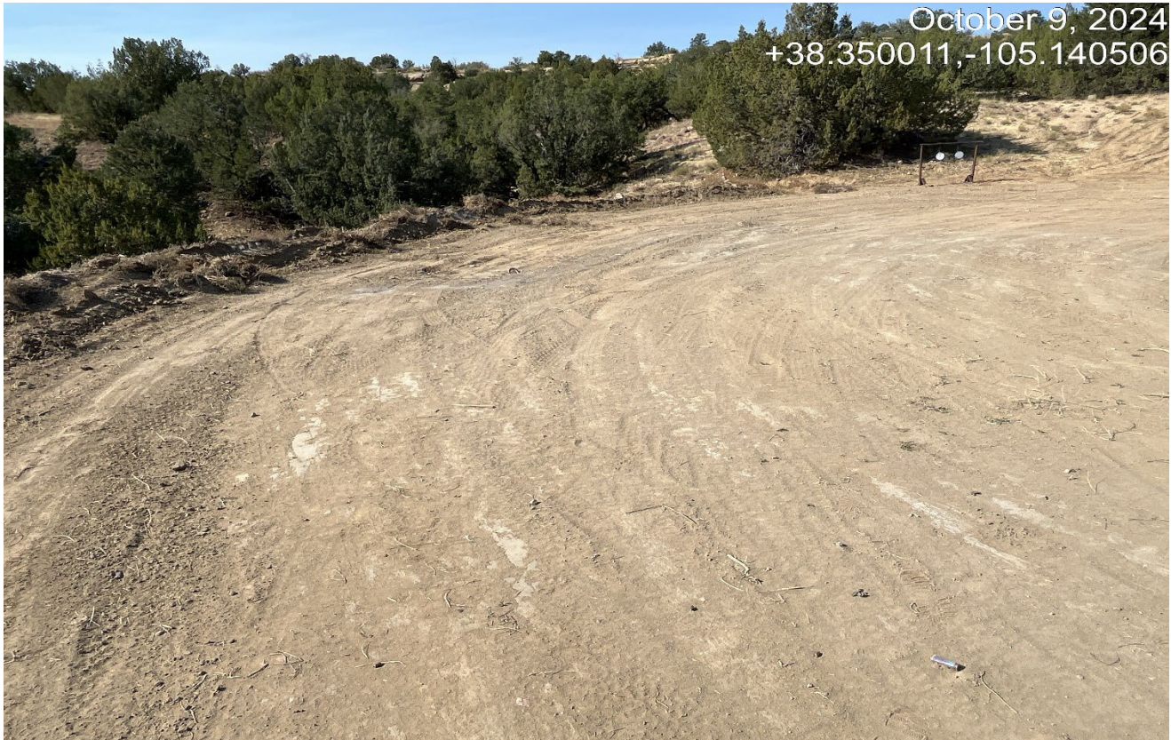
Photo 12. The drill cutting pile has been removed but there is still grey material present since the cuttings were not stored in a liner.
