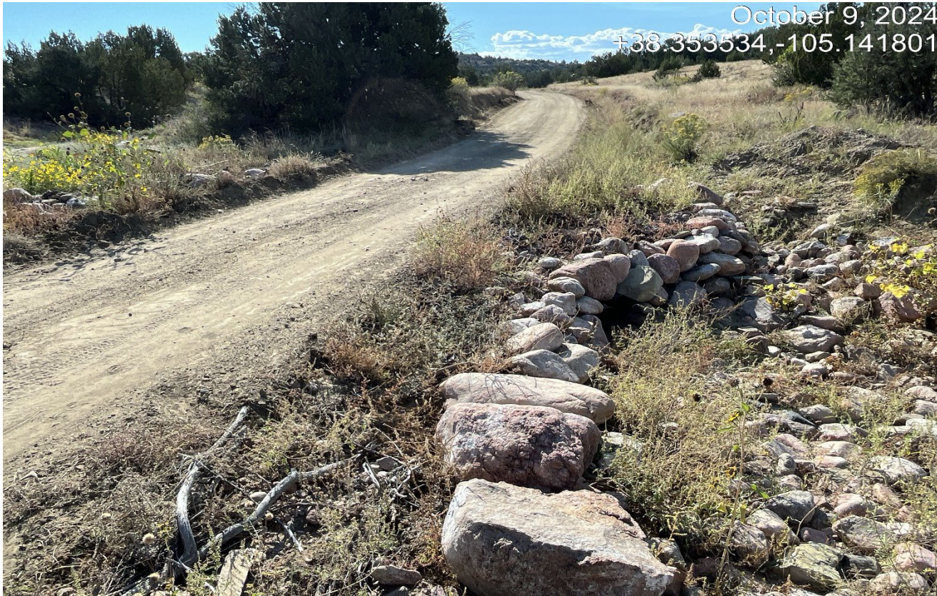
Photo 2. Facing toward the intermittent drainage that had washed out the road. There are two 1' culverts installed which may not be adequately sized for heavy storm events. The road rock used for outlet protection could become easily displaced.
