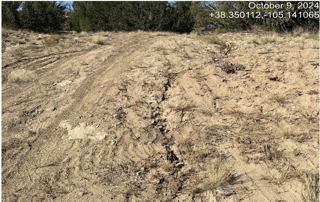
Photo 16. Facing toward the cut slope at the southwest side of the location. There are signs of erosion and the cut slope is not stabilized with vegetation.
