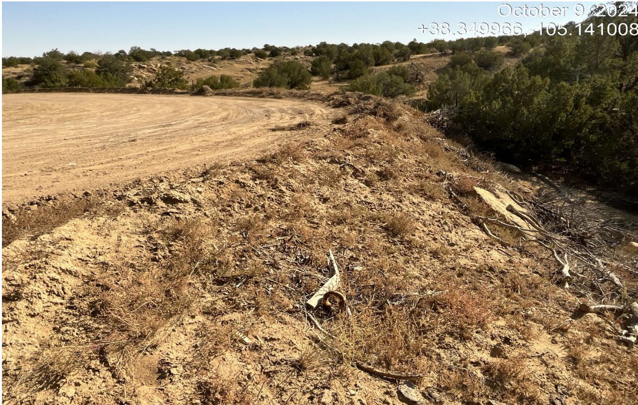
Photo 15. Facing toward the fill slope at the south side of the location which consists of weeds and is not stabilized.
