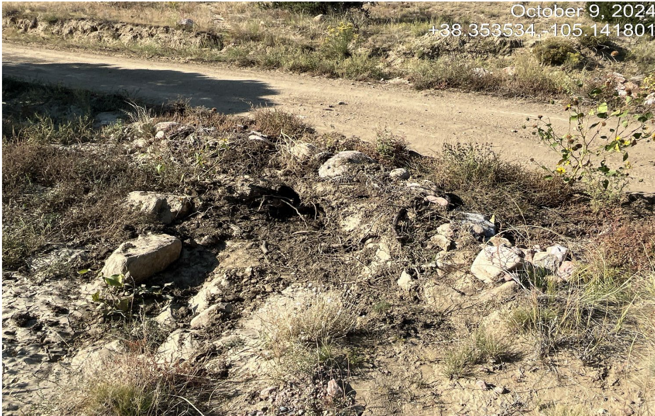
Photo 3. Facing toward the intermittent drainage that had washed out the road. There are two 1' culverts installed which may not be adequately sized for heavy storm events. The culvert has already filled up with debris and it appears debris was washed over the road. The culverts are insufficiently sized.
