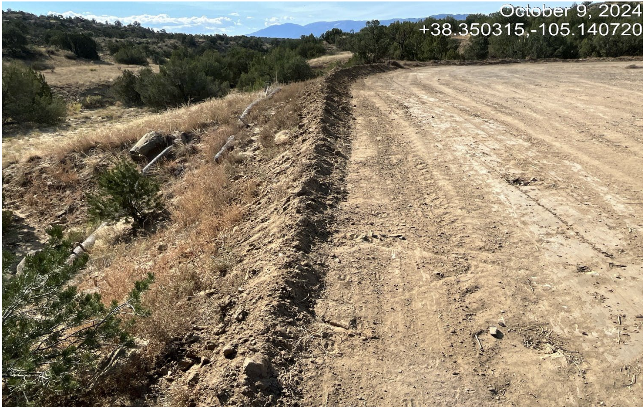
Photo 11. Facing southwest toward the fill slope of the location. There are loose soils pushed out along the edge of the pad that can erode offsite.
