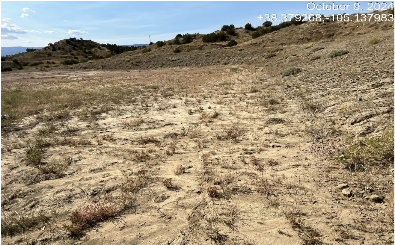
Photo 8. Facing south along the cut slope. There are rilling erosion along the cut slope which is not stabilized.
