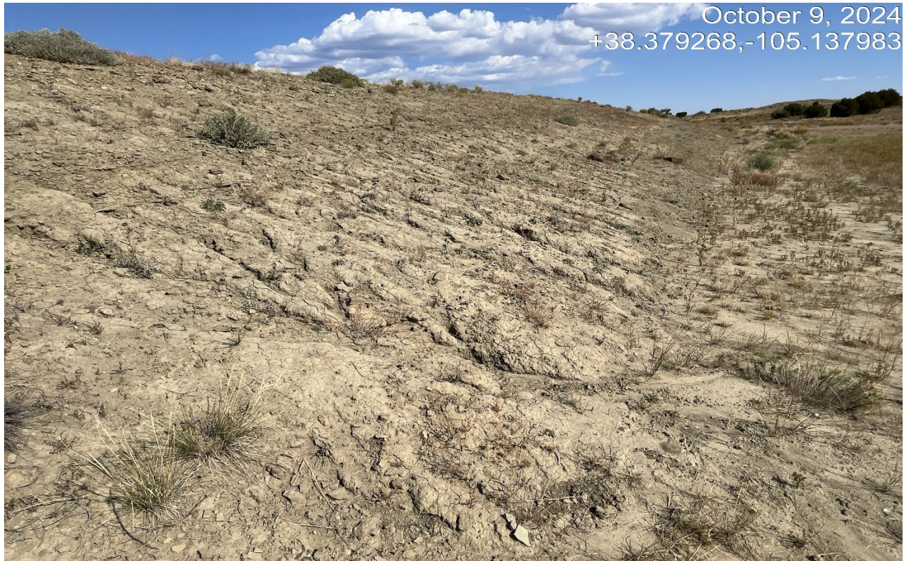
Photo 9. Facing northwest along the cut slope. There cut slope is not stabilized.
