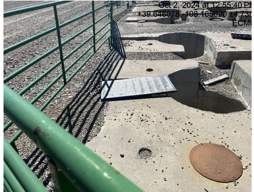
Debris (screen from drilling rig shakers) and open holes
