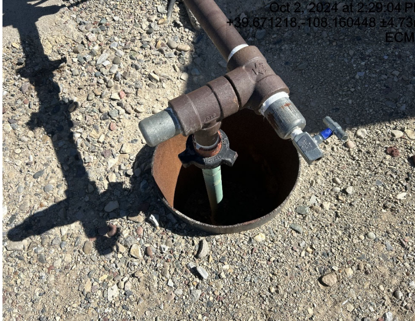
Open holes at well heads
