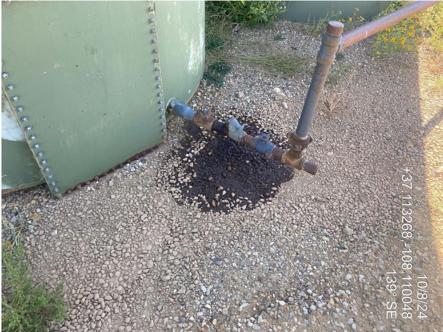
Photo 5. View of impacted surface material with the tank secondary containment/berm.
