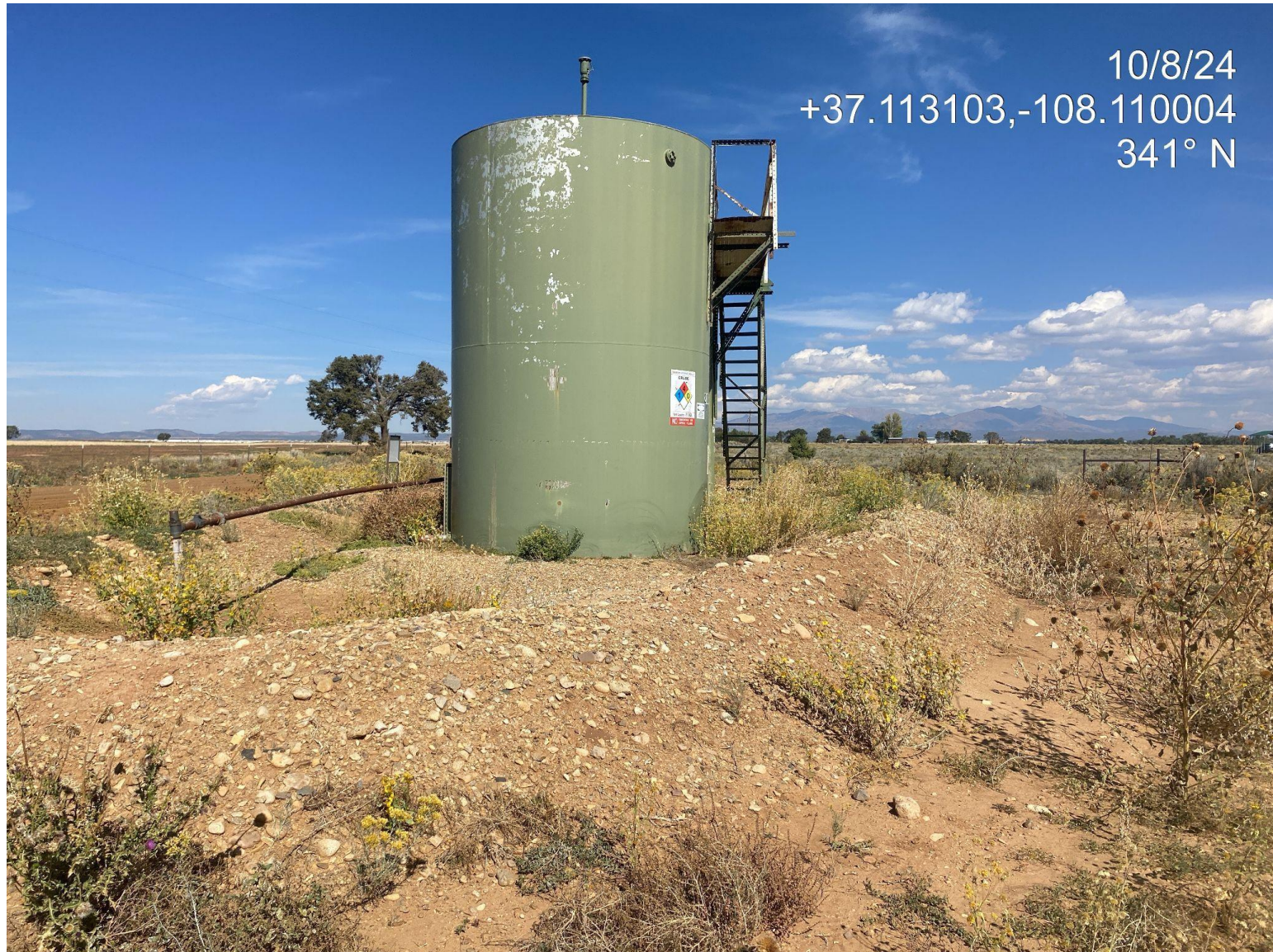
Photo 4. View of weedy debris/vegetation encroaching/over taking tank berm which is affecting permeability.
