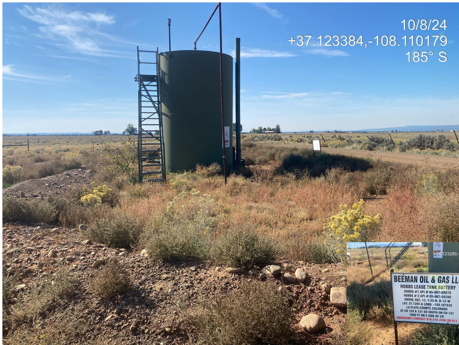
Photo 3. View of Hubbs 1 and 2 associated tank battery. Note: Weedy Russian Thistle debris are encroaching on tank berm and affecting berm integrity.
