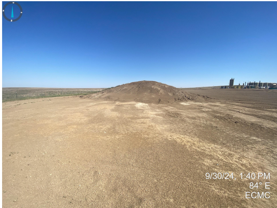
Photos 13 & 14. It appears that topsoil has been removed from the existing stockpile area (western side).
