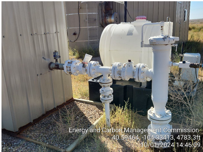
Photo 7 – Gas Sales Line LOTO Downstream of Meter
