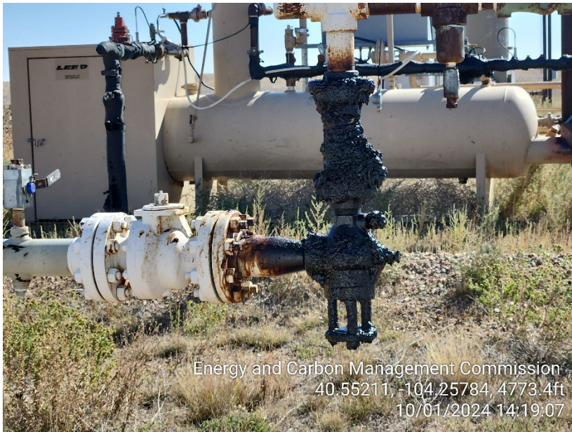
Photo 11 – Rupture Pin Valve leaking
