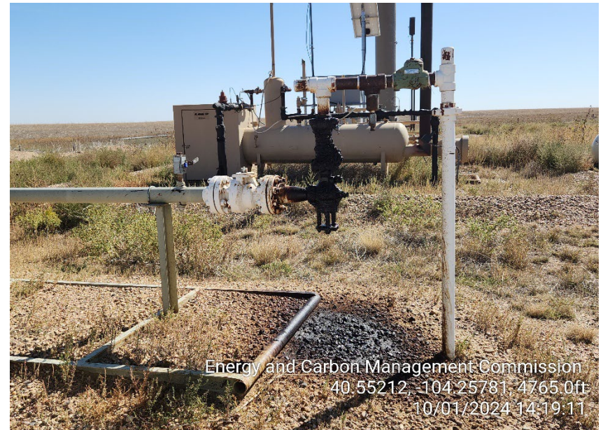
Photo 12 – Stained Soil at Rupture Pin Valve
