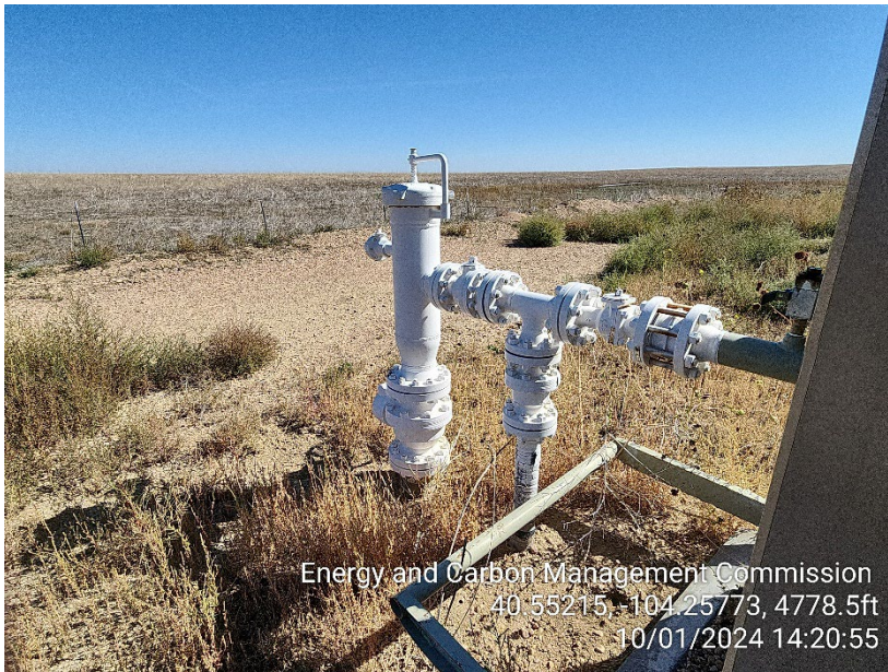
Photo 15 – Valves open downstream of Meter
