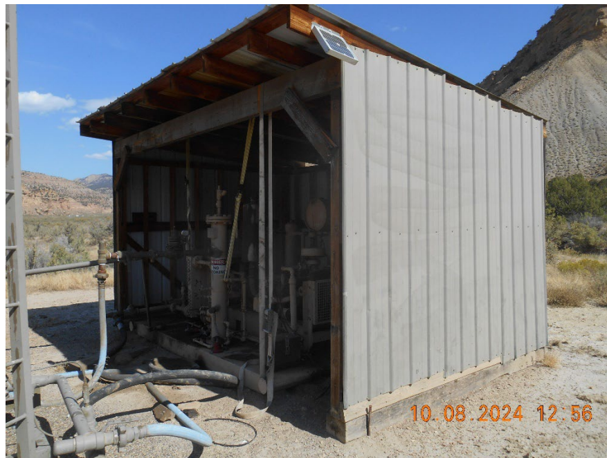
Compressor inside housing
