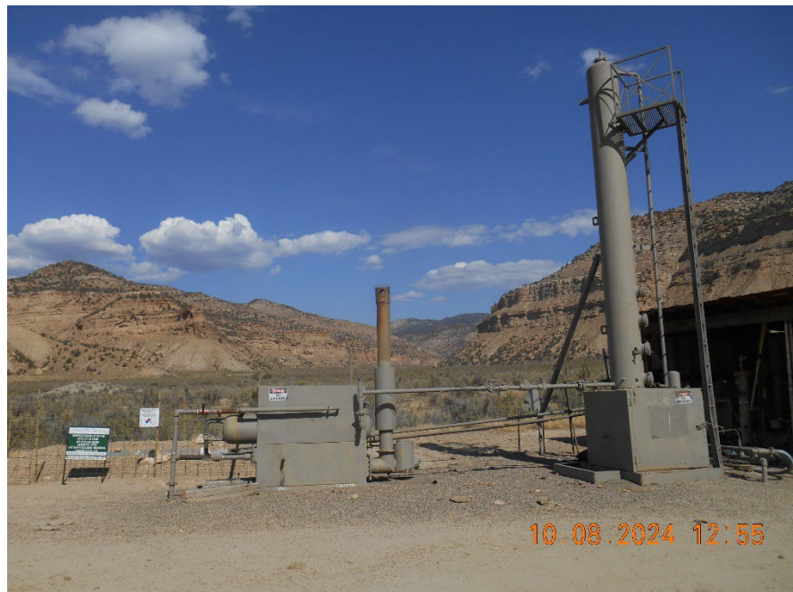
Separator and Dehydrator
