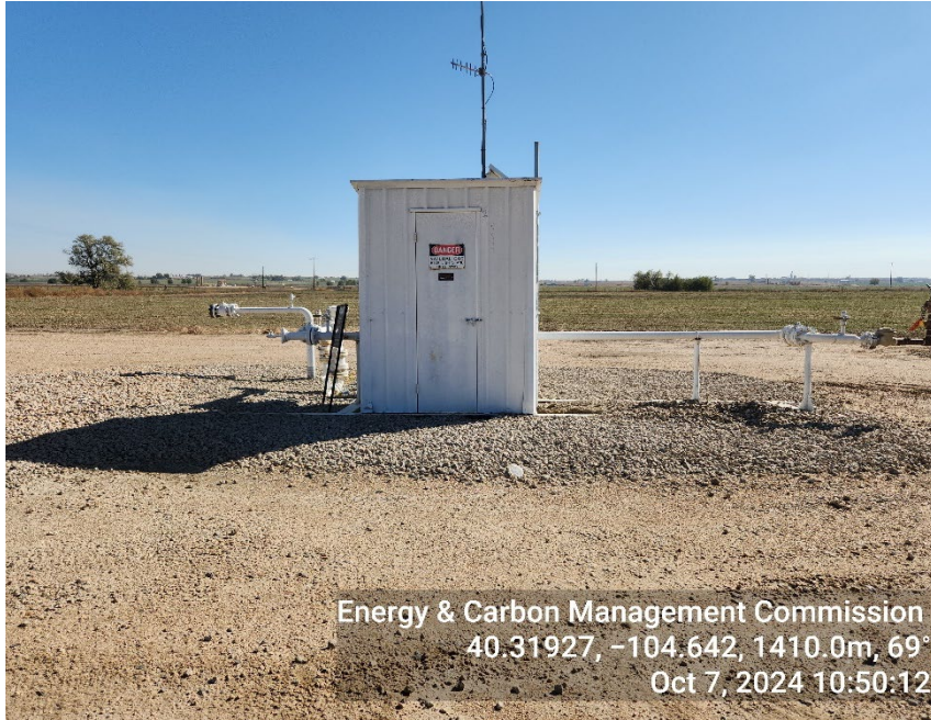
Photo 3: Unused/disconnected gas meter
