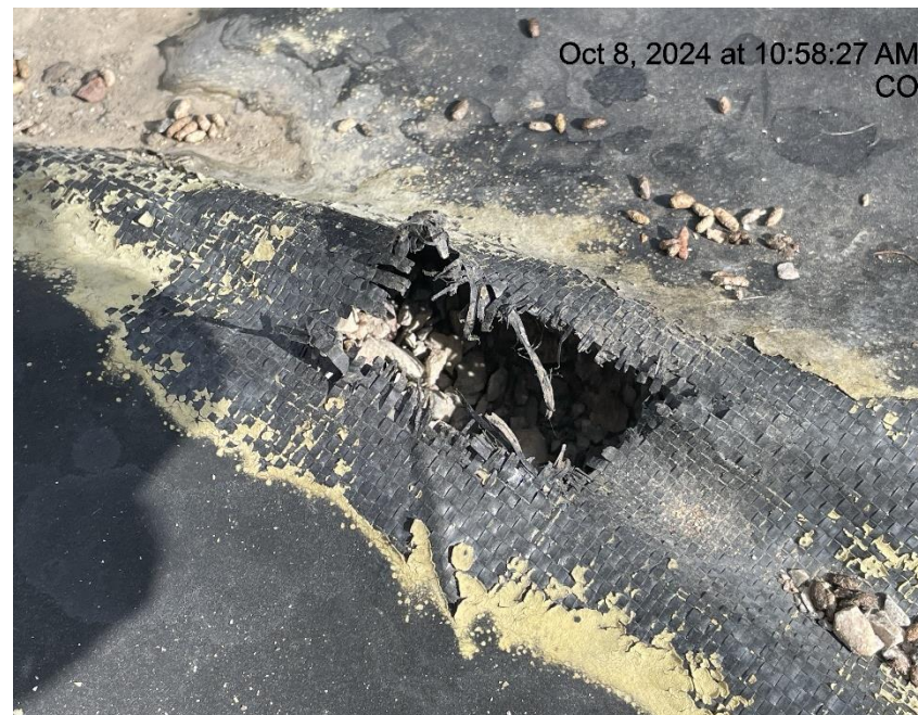
Photo # 3863 Hole in secondary containment liner/liner needs maintenance
