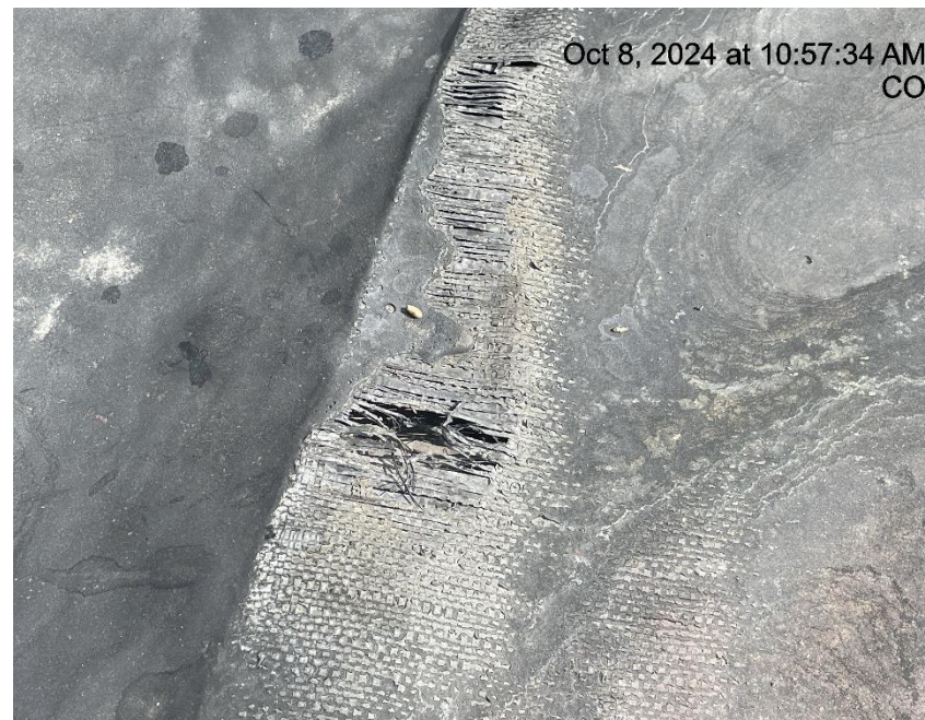
Photo # 3865 Hole in secondary containment liner/liner needs maintenance
