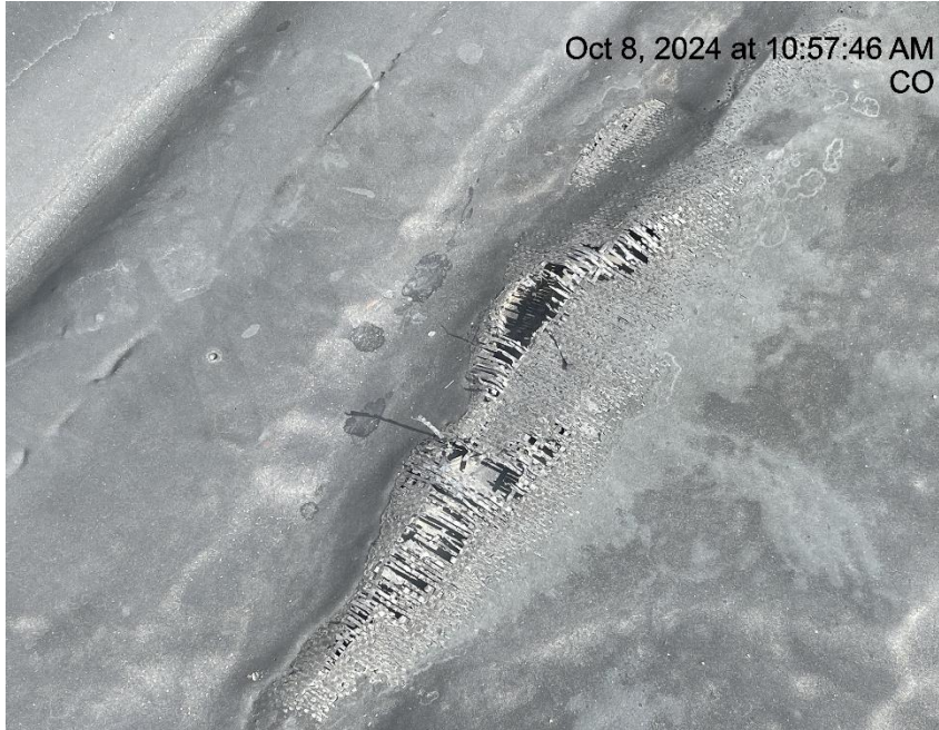
Photo # 3866 Hole in secondary containment liner/liner needs maintenance
