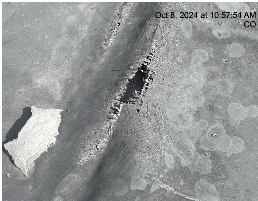
Photo # 3864 Hole in secondary containment liner/liner needs maintenance
