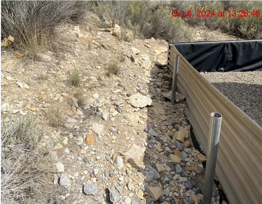
Insufficient Erosion Control – Photo #04034
