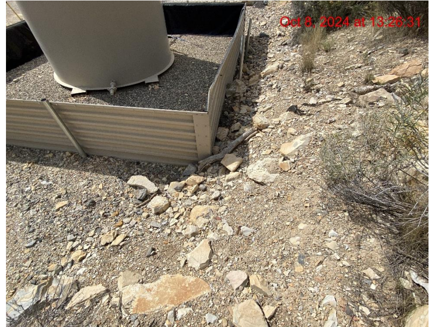
Insufficient Erosion Control – Photo #04033
