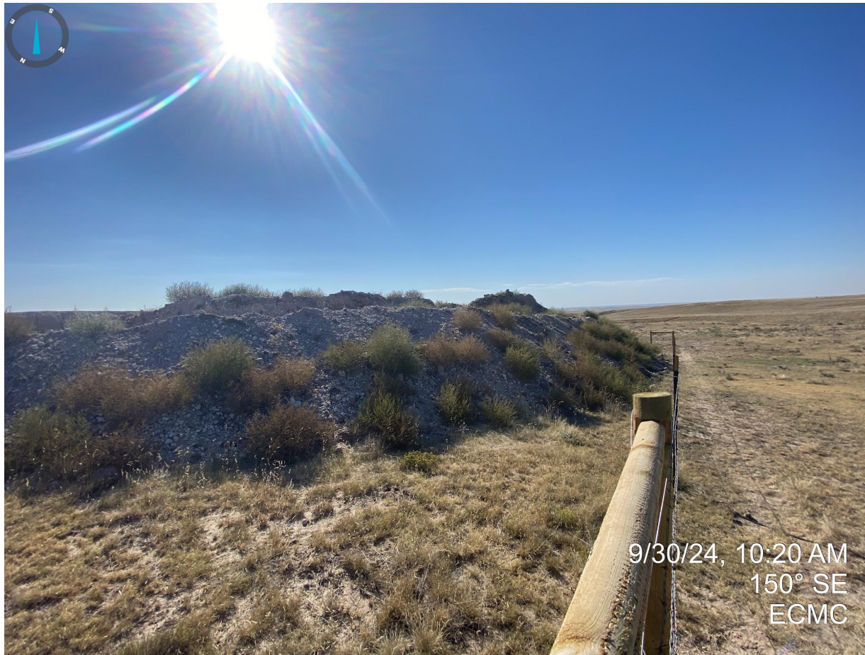
Photo 7. Taken from the north side of the stockpiled soils. No perimeter stormwater control measures/BMPs, or impermeable liners underneath the stockpile were observed during this inspection. Impacted soils appear to have been placed directly on top of undisturbed lands. Additionally, it does not appear that topsoil has been salvaged Per Rule 1002.b prior to stockpiling the soil on undisturbed portions of land. Undesirable vegetation observed throughout stockpiled areas.
