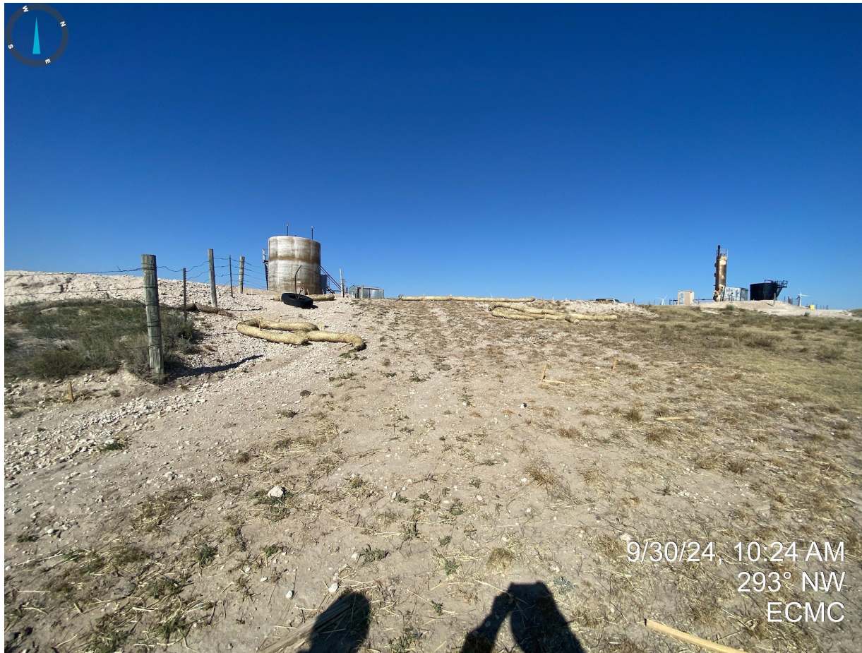
Photo 14. Erosion degradation occurring on the northern/eastern portion of the production areas, near the pit; stormwater control measures remain inadequate as they are not properly installed.
