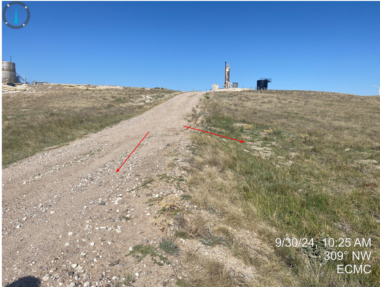
Photo 6. Sediment deposition and erosion degradation along the access road, east of pit.
