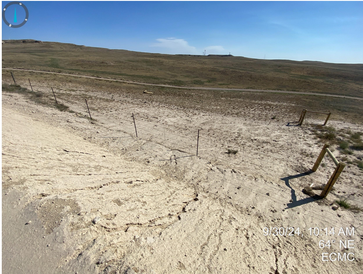
Photo 18. Erosion degradation on the eastern pit walls. This portion of the pit wall was recently repaired and is still experiencing erosion issues; soils remain unstabilized.
