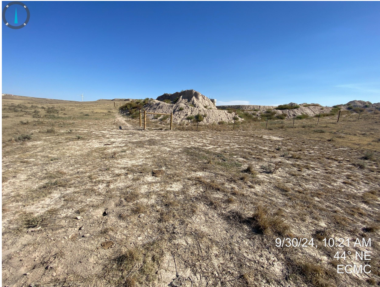
Photo 9. Sediment deposition resulting from unstabilized stockpiles, southwest corner of the pit.
