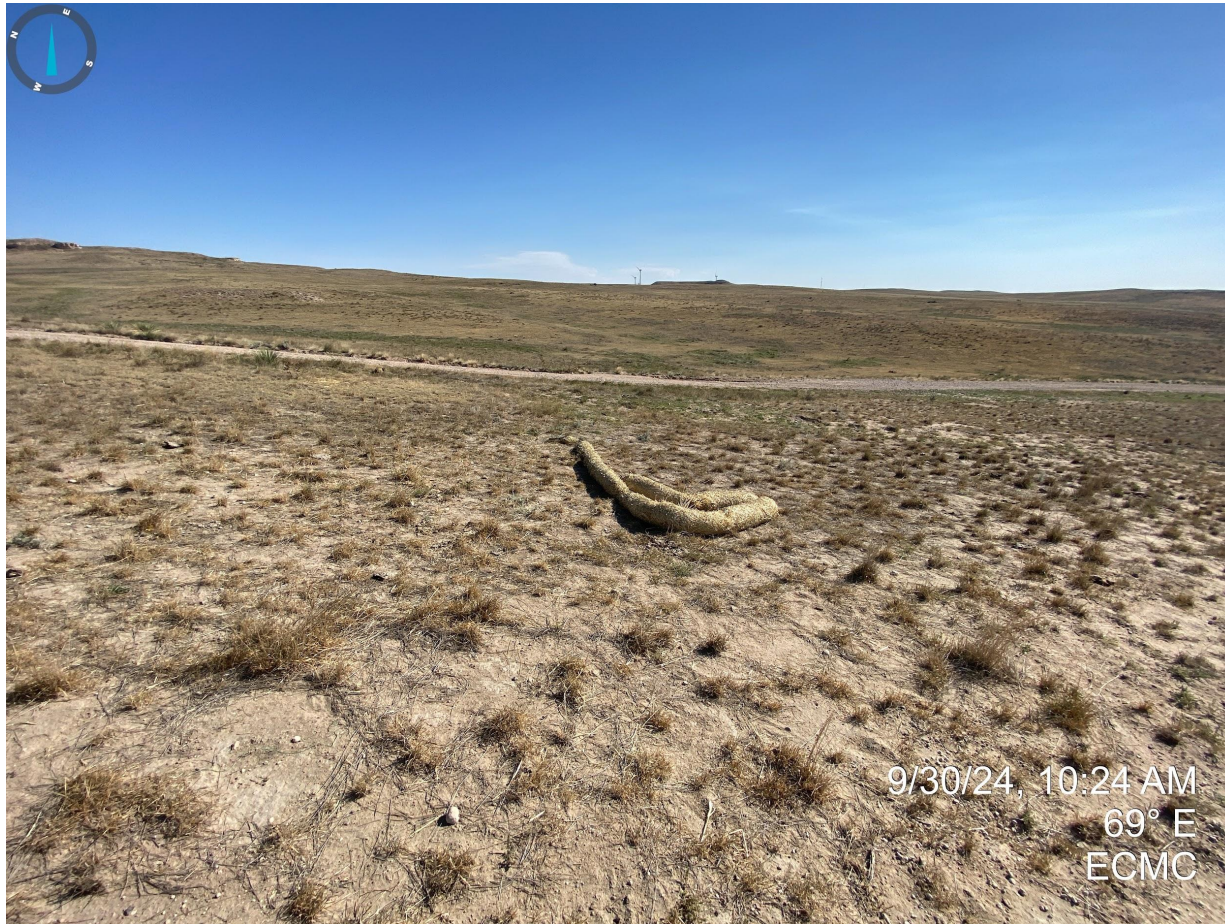
Photo 15. Straw wattle observed east of pit needs to be removed or reinstalled.
