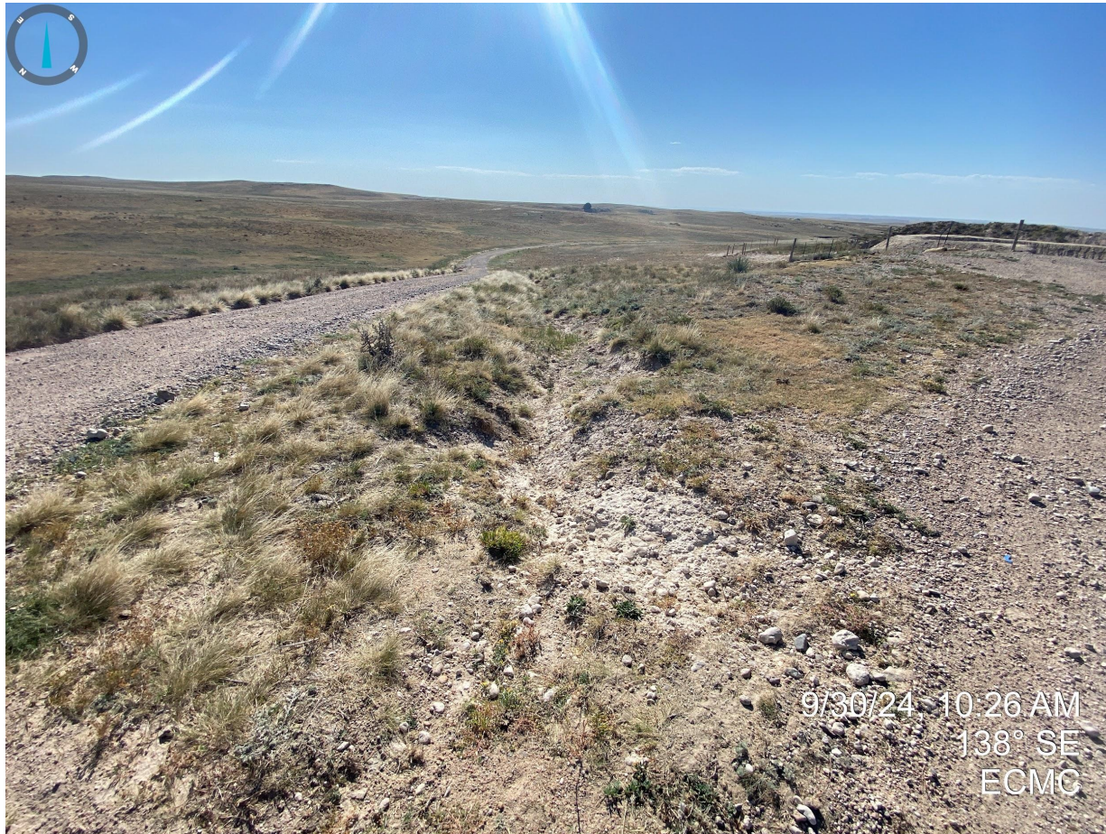
Photo 2. Taken north of pit. Evidence of erosion degradation, previously documented, does not appear to have been repaired/stabilized with no evidence of control measures/BMPs observed that would prevent further erosion of the production areas and access roads.
