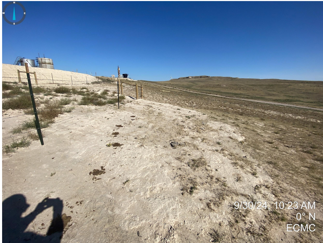
Photo 12. Sediment deposition resulting from unstabilized soils, southeast corner of the pit.
