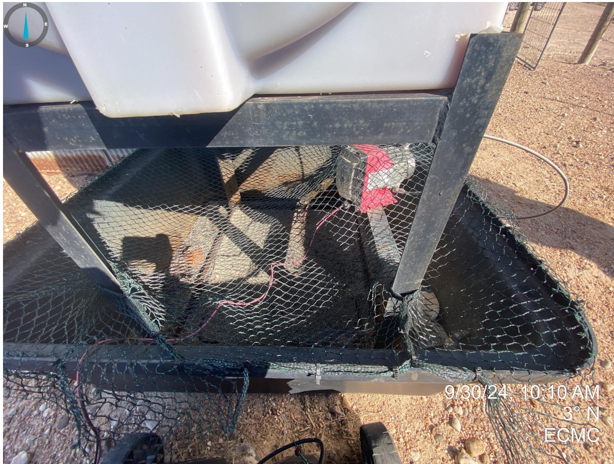
Photo 1. Free fluids appear to have been removed from the secondary containment at day tank.
