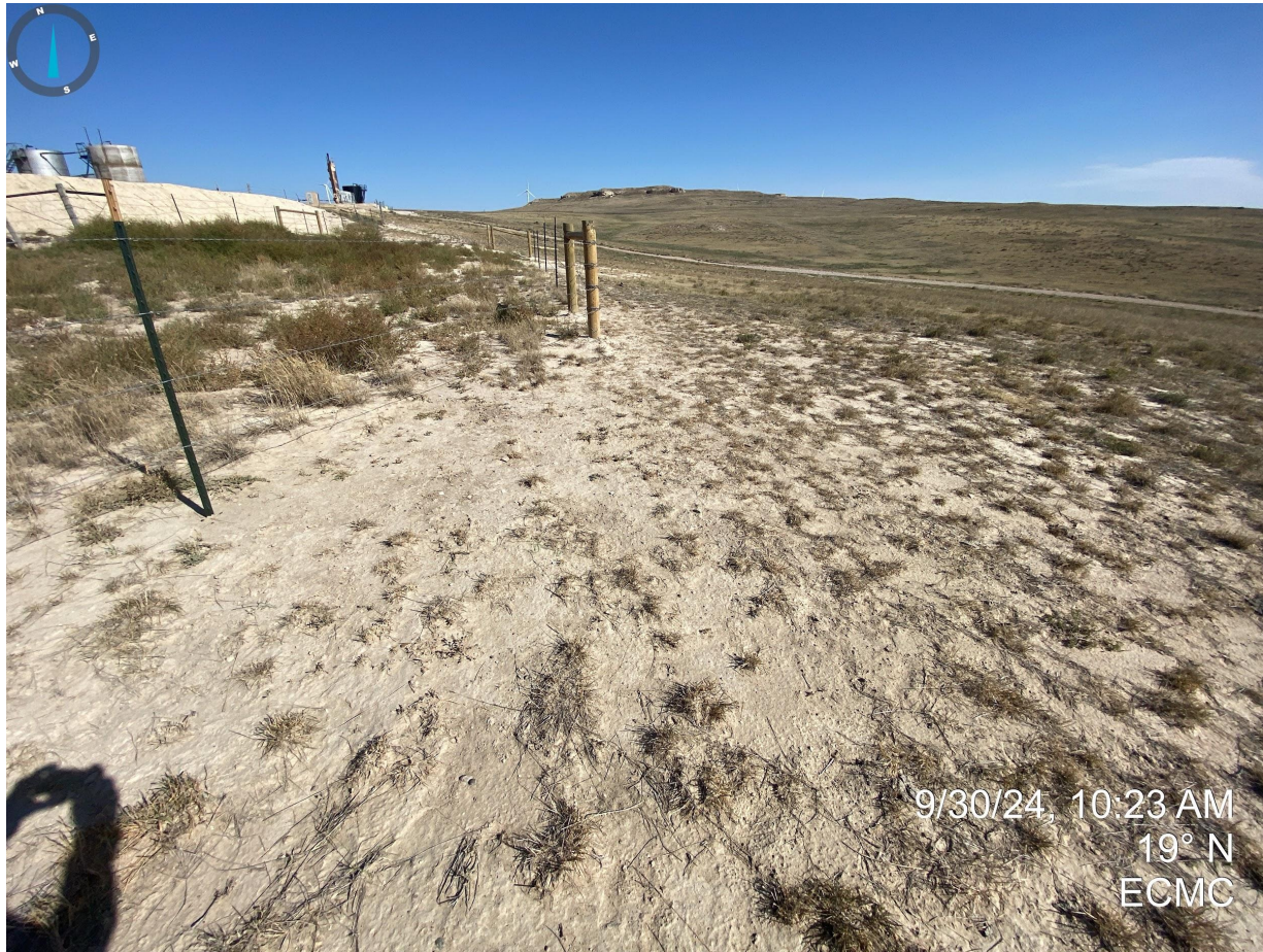
Photo 11. Taken southeast of the excavated area and stockpiled material; no apparent perimeter stormwater control measures and sediment deposition observed.
