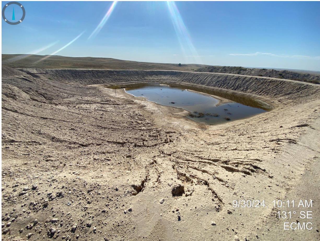
Photo 16. Erosion degradation observed within pit walls.
