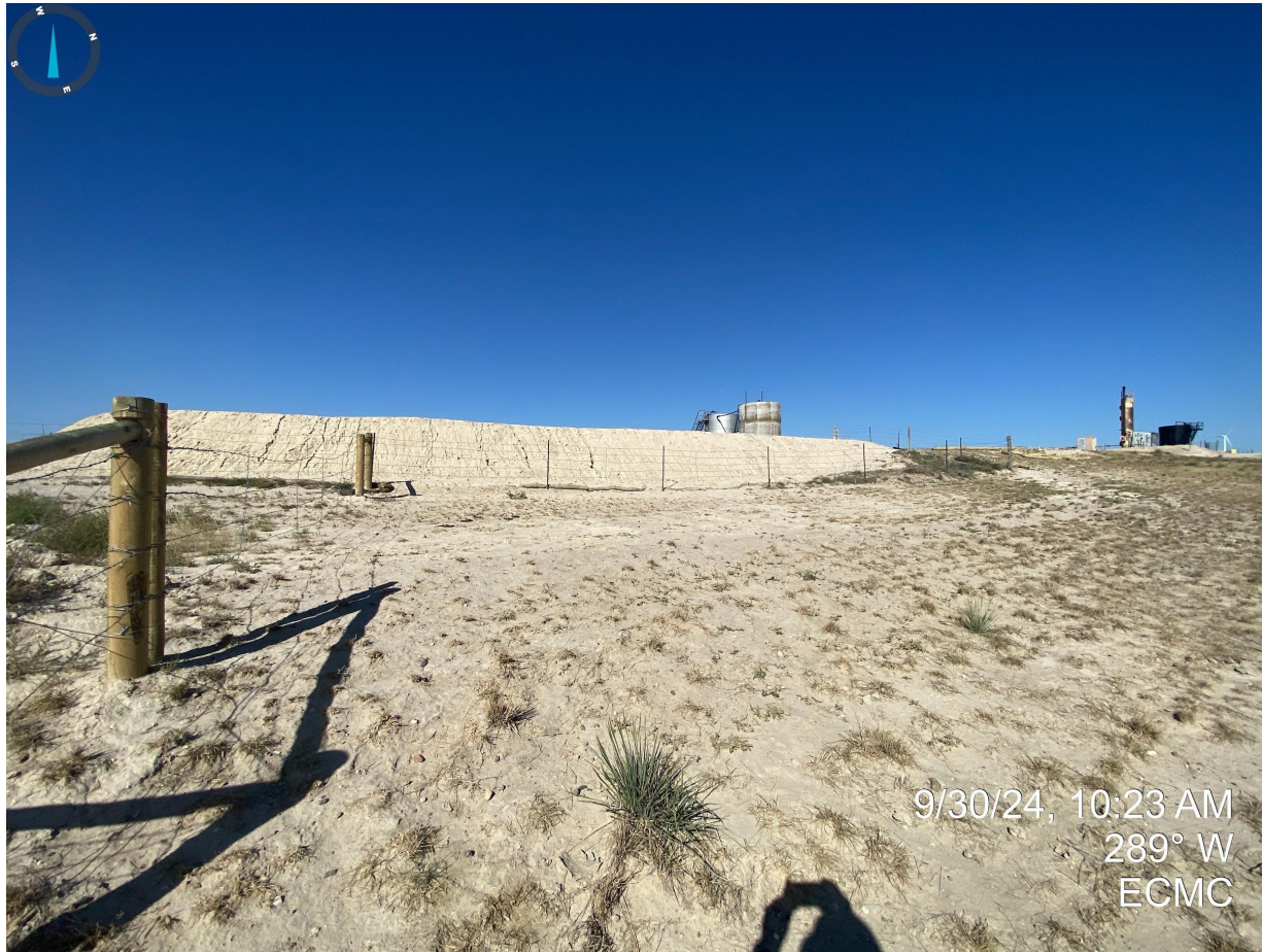
Photo 13. Sediment deposition resulting from unstabilized soils, eastern portion of the pit. Stormwater control measures remain inadequate.
