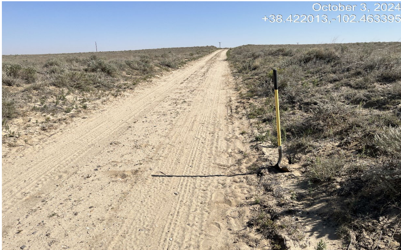
Photo 2. Facing east along the main access road. The road is below the grade of the land and causes issues with snow accumulation during the winter.
