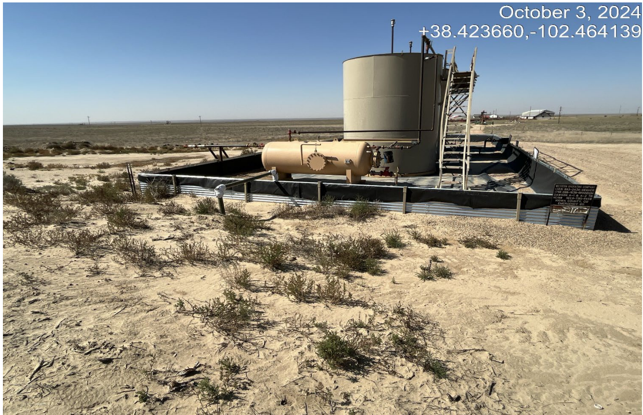
Photo 3. Facing east at the tank battery. Tanks have been installed with secondary containment.
