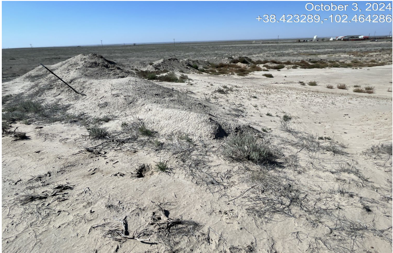
Photo 5. Facing toward the stockpile of soil which remains bare and susceptible to erosion.
