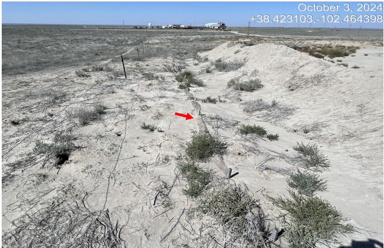
Photo 6. Facing east at the south side of the tank battery. It appears the stock piled soils have wind blown and almost completely covered up the perimeter wattles shown at red arrow.
