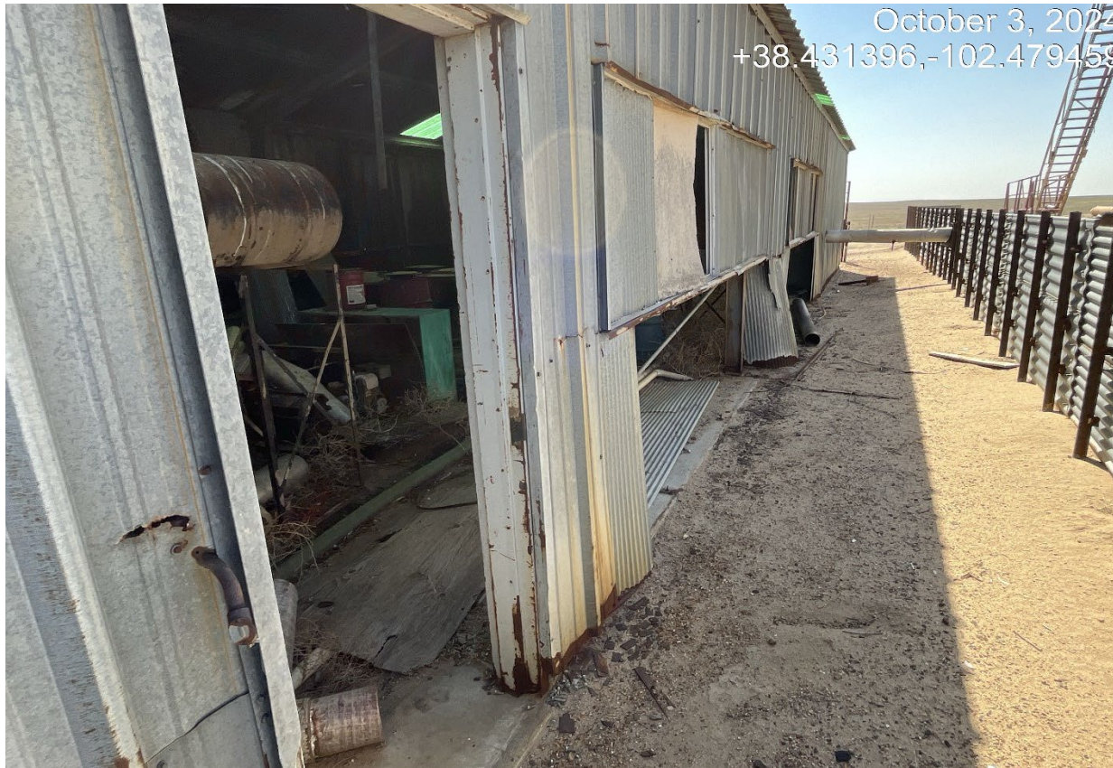
Photo 3. There was pieces of tin rattling and loose along the back side of the storage shed.
