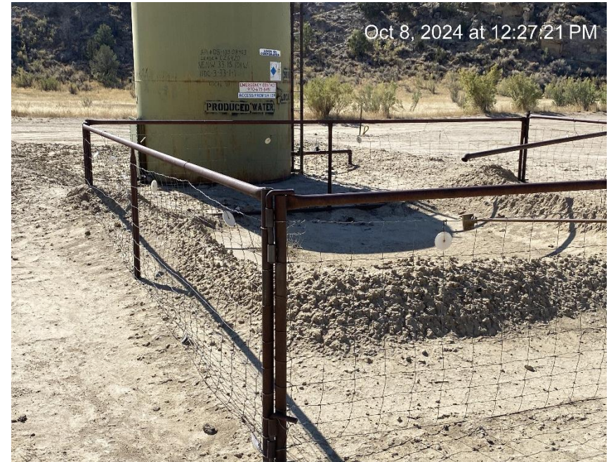
Inadequate tank berm
