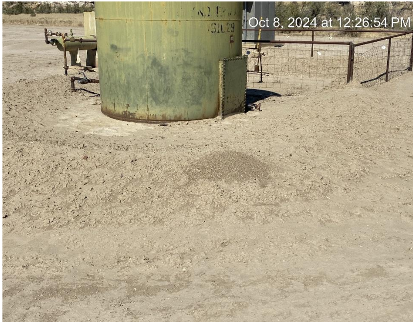
Inadequate tank berm
