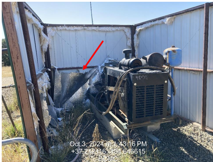
Photo 3 – Sound Panels, Insulation is dilapidated
