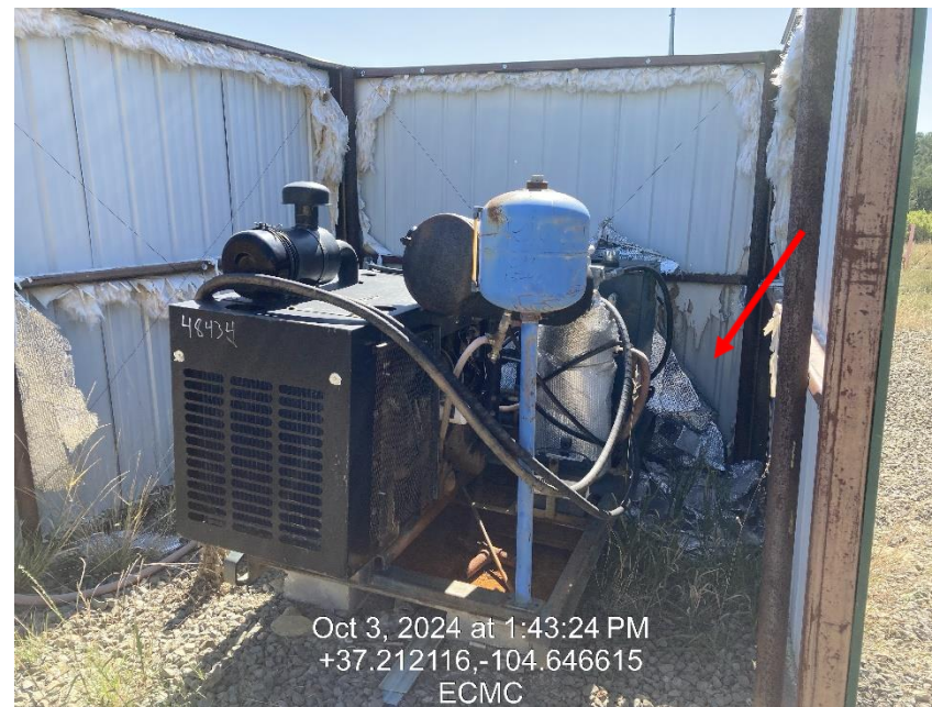
Photo 4 – Sound Panels, Insulation is dilapidated
