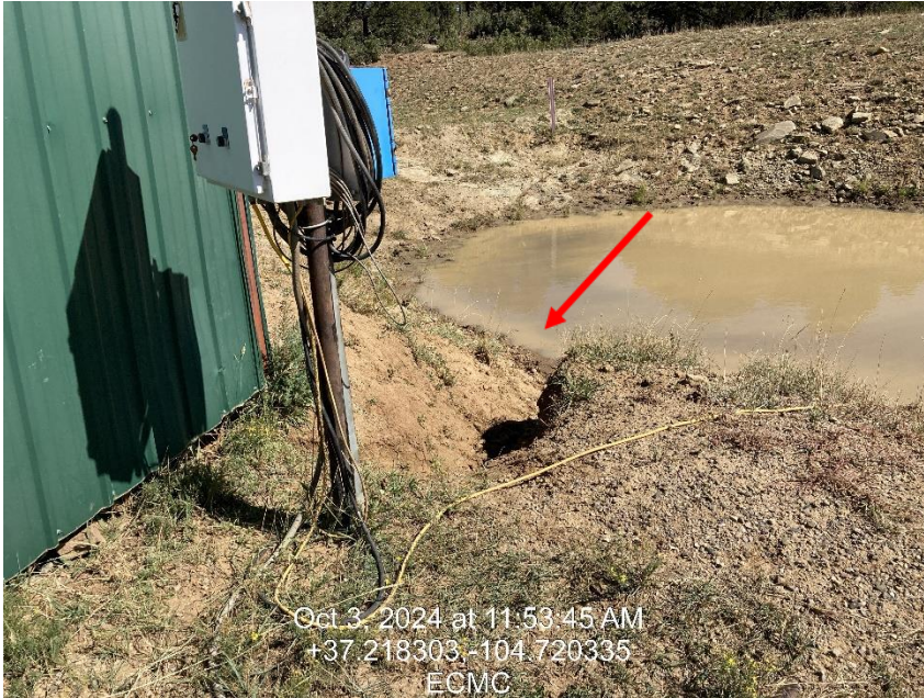
Photo 5 – Stormwater entering pit
