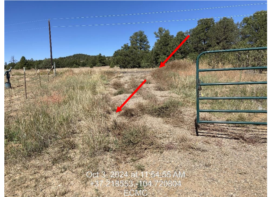
Photo 6 – Erosion and Undesirable weeds along access road
