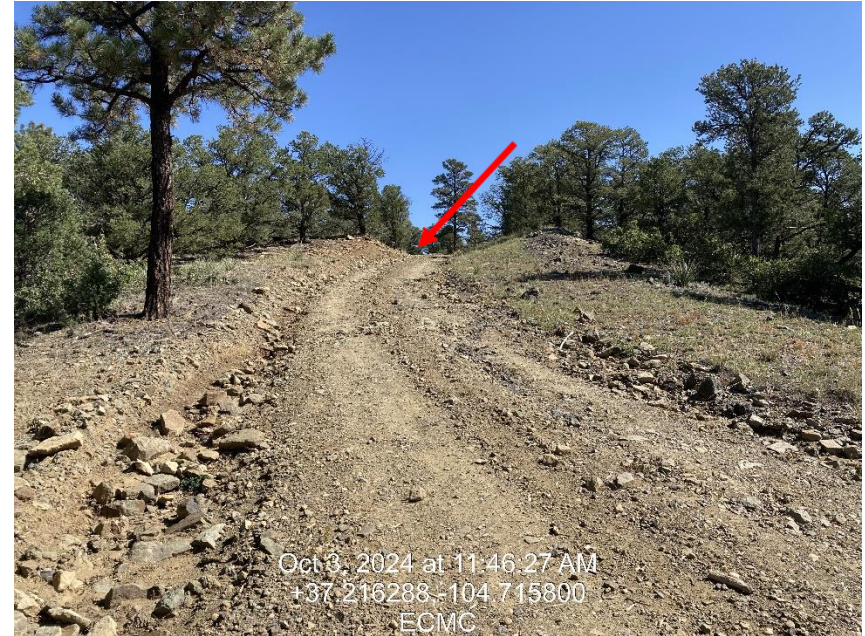
Photo 8 – Erosion along access road
