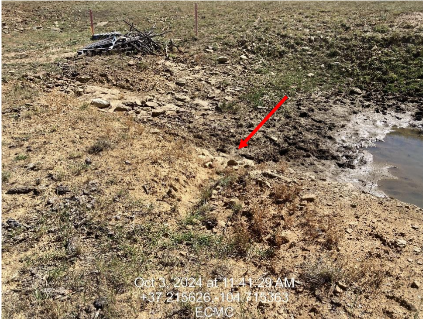
Photo 7 – Pit Facility ID 301072, Stormwater entering pit
