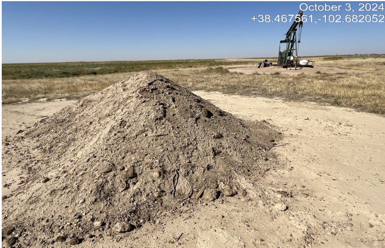
Photo 7. There is a pile of oily contaminated soil material stored on location that must be removed and properly disposed. Previous CA was not completed.
