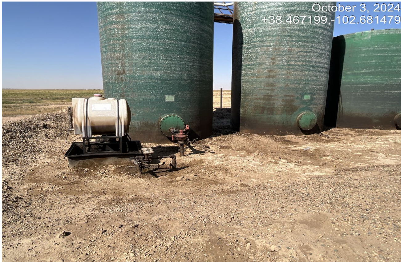
Photo 3. There are stained soils at the back side of the tank battery that must be cleaned up. Previous CA was not completed.
