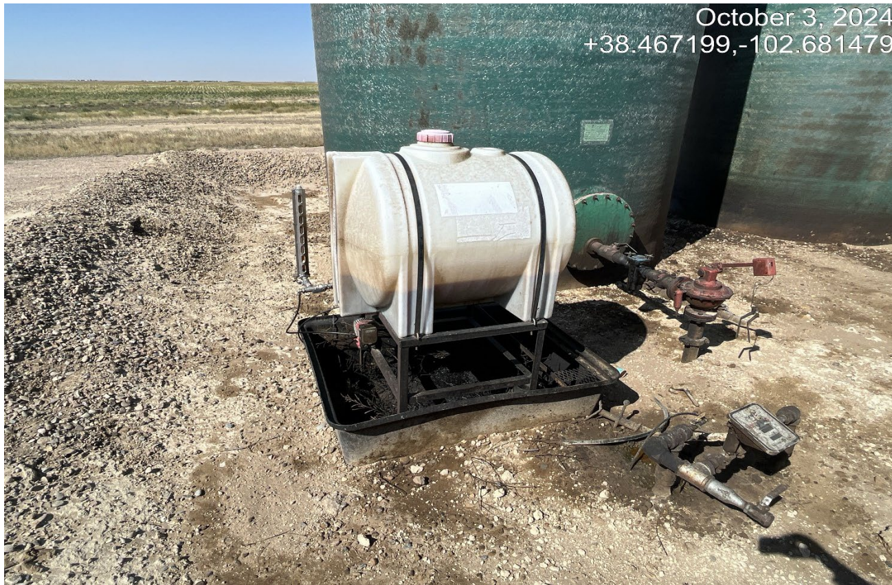
Photo 4. There is oily material inside the black containment which has no wildlife protections. There are stained soils around the tank battery that must be cleaned up. Previous CA was not completed.
