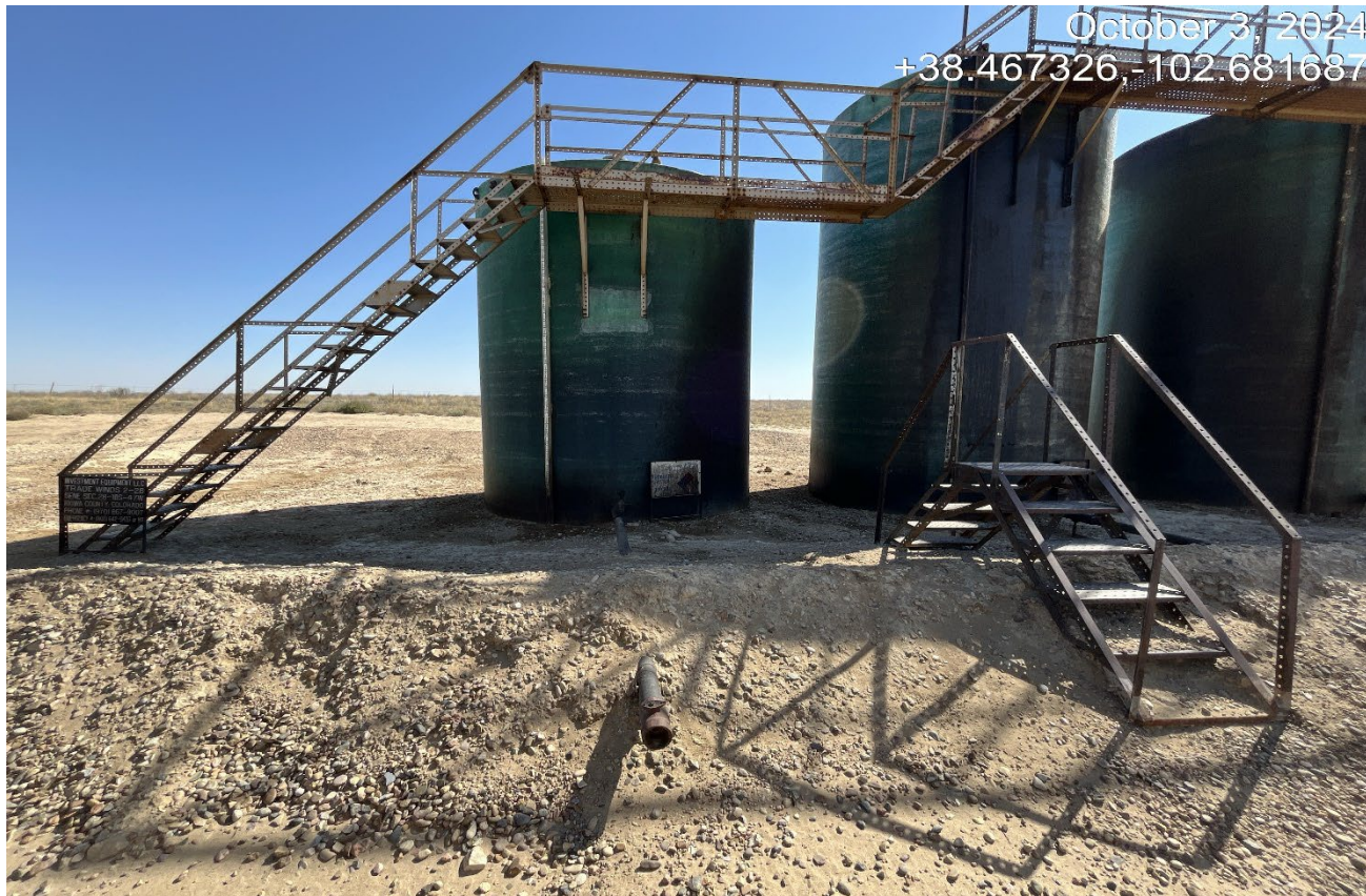
Photo 2. Facing toward the tank battery. The H 2 S wind sock is missing. There is oily stained soils that extend the entire area of the containment from a previous spill that was never cleaned up. Previous CA's were not completed.
