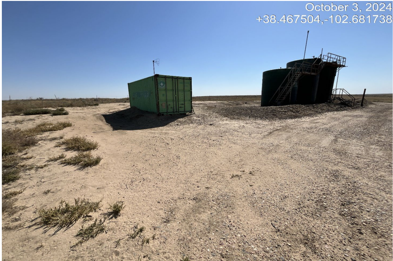
Photo 1. Facing southeast toward the location. The soils around the conex have eroded and no BMP's have been installed. The H2S wind sock is missing. Previous CA's were not completed.
