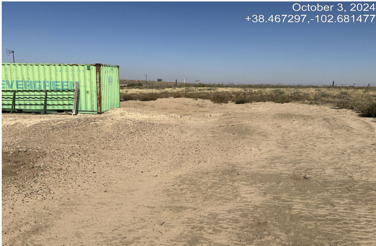
Photo 6. Facing north at the east side of the location. The soil near the conex have eroded and are bare of vegetation. This area must be stabilized to prevent further erosion.
