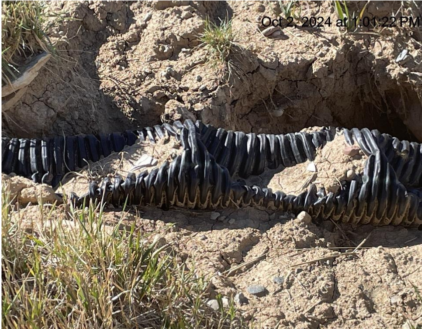
Photo # 3382 Drain line showing signs of damage
