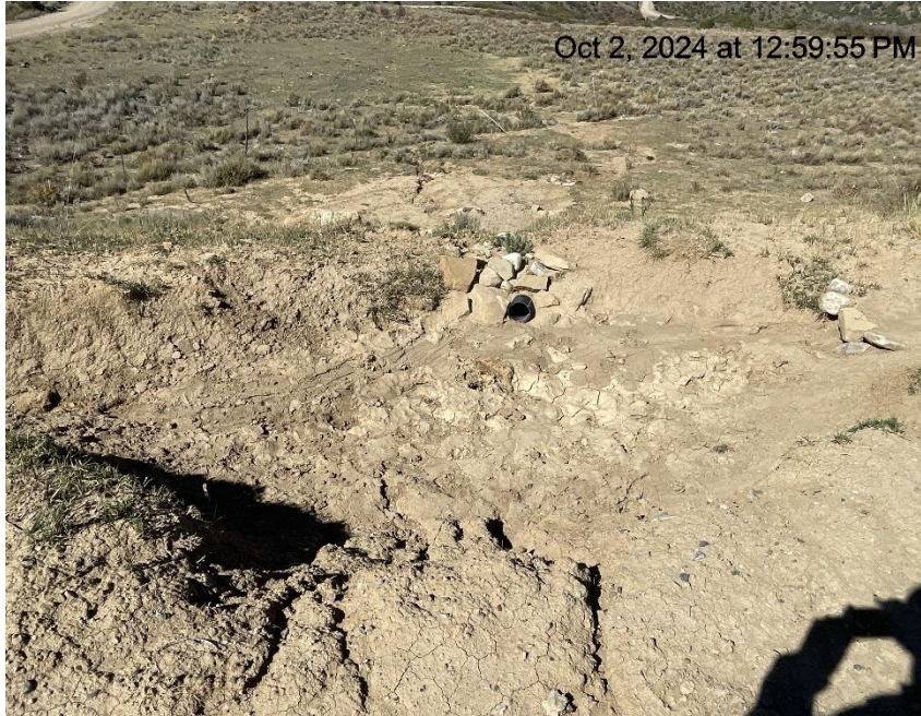
Photo # 3378 Sediment trap needs maintenance/large amount of sediment in catch basin/sediment laden stormwater entering drain & being carried off location
