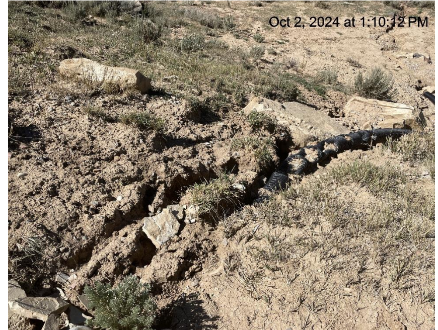
Photo # 3381 Erosion & sediment transport on slope near drain line
