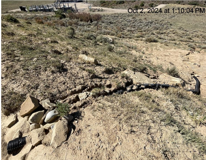
Photo # 3380 Erosion & sediment transport on slope near drain line
