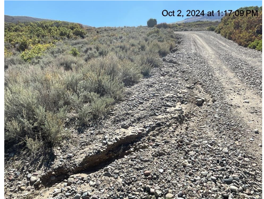
Photo # 3385 Ditch along lease road needs maintenance
