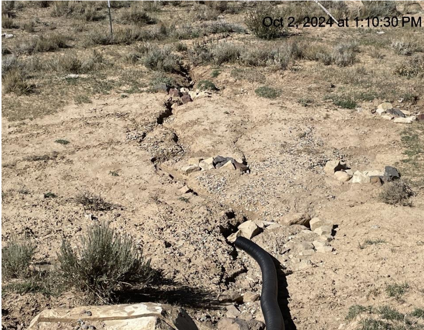
Photo # 3384 Erosion & sediment transport at drain line outlet/BMP's need maintenance
