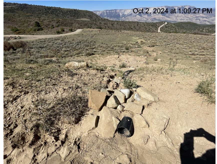
Photo # 3379 Sediment trap needs maintenance/large amount of sediment in catch basin/sediment laden stormwater entering drain & being carried off location
