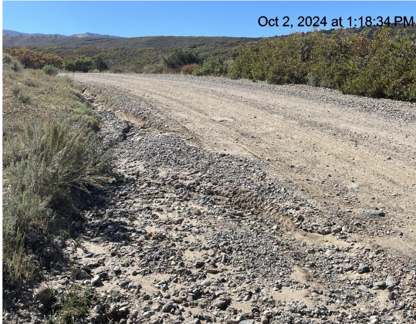
Photo # 3386 Ditch along lease road needs maintenance
