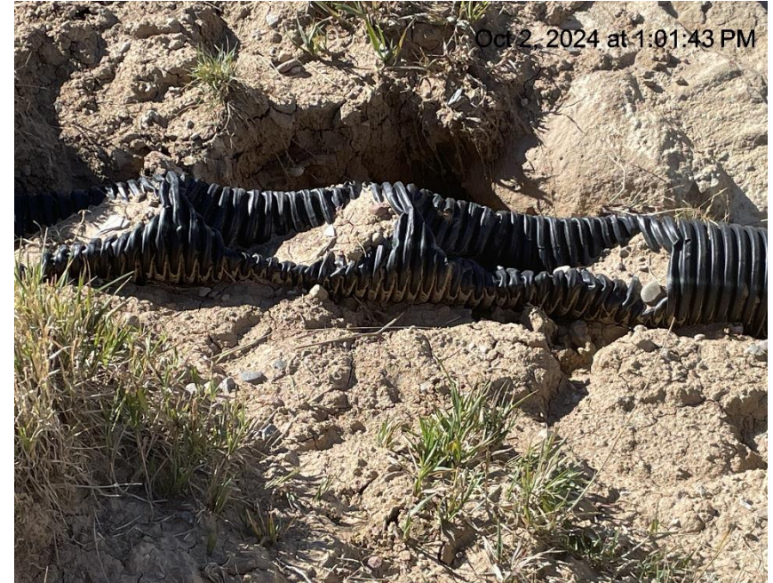
Photo # 3383 Drain line showing signs of damage
