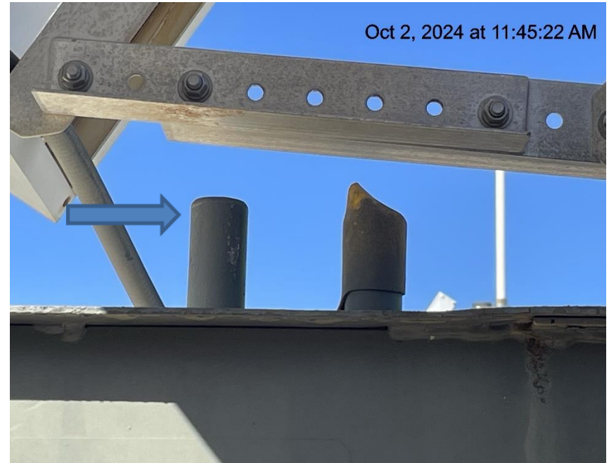
Photo # 3072 PRV vent line does not comply with CECMC pressure safety device rules
