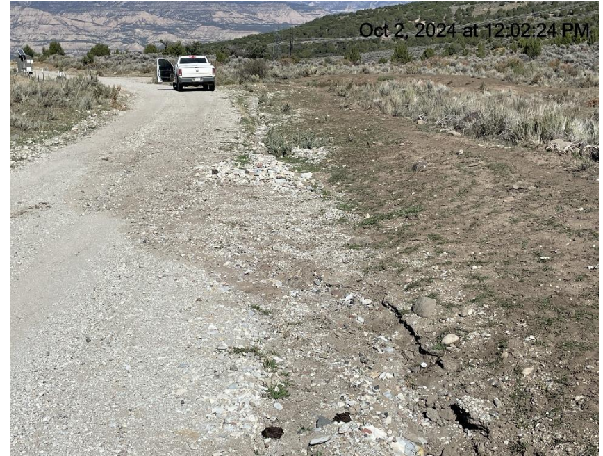
Photo # 3074 Ditch needs maintenance/ditch is full of sediment & sediment is being transported onto the lease road (on lease road approximately 1/10 th to 2/10 th of a mile from location)
