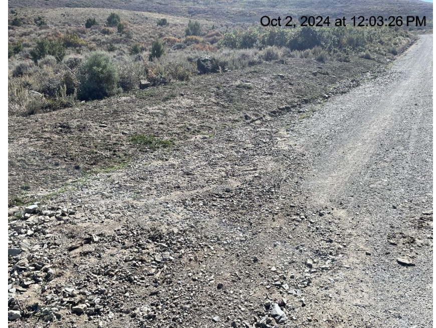
Photo # 3076 Ditch needs maintenance/ditch is full of sediment & sediment is being transported onto the lease road (on lease road approximately 1/10th to 2/10th of a mile from location)
