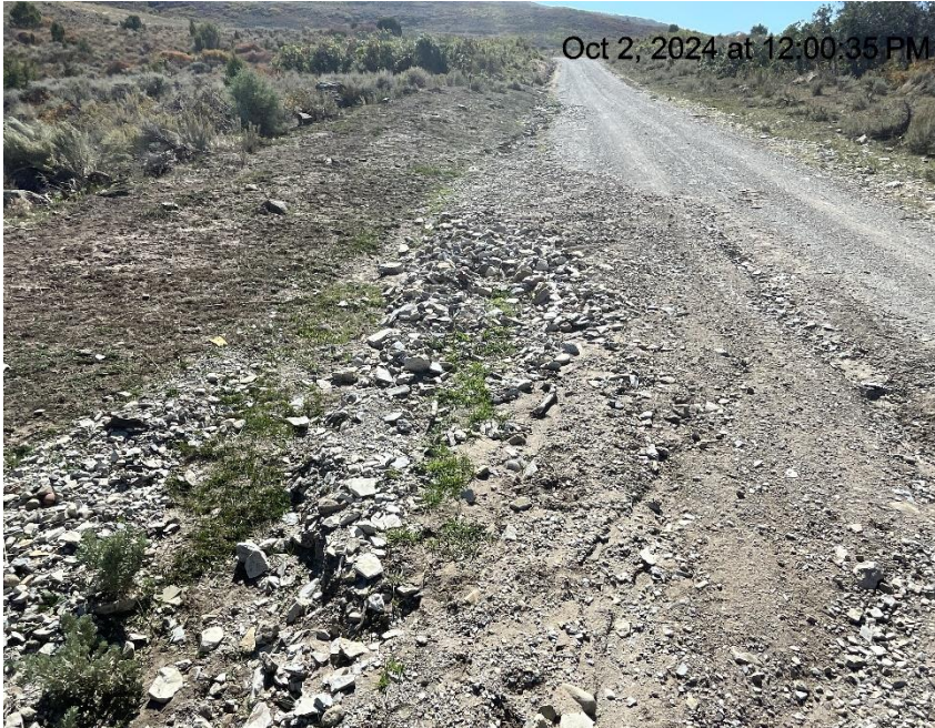
Photo # 3073 Ditch needs maintenance/ditch is full of sediment & sediment is being transported onto the lease road (on lease road approximately 1/10 th to 2/10 th of a mile from location)
