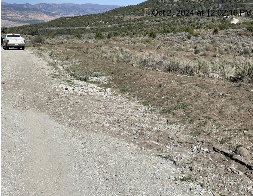
Photo # 3075 Ditch needs maintenance/ditch is full of sediment & sediment is being transported onto the lease road (on lease road approximately 1/10th to 2/10th of a mile from location)
