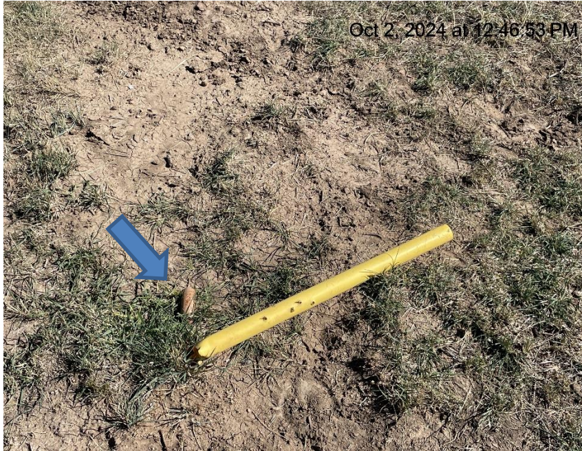
Photo # 3271 Improperly marked deadman
