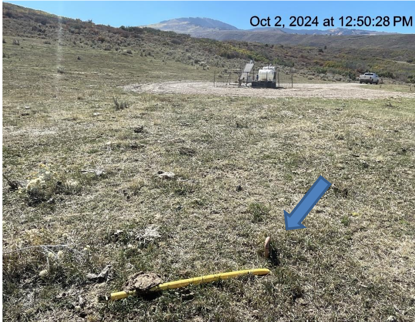
Photo # 3273 Improperly marked deadman
