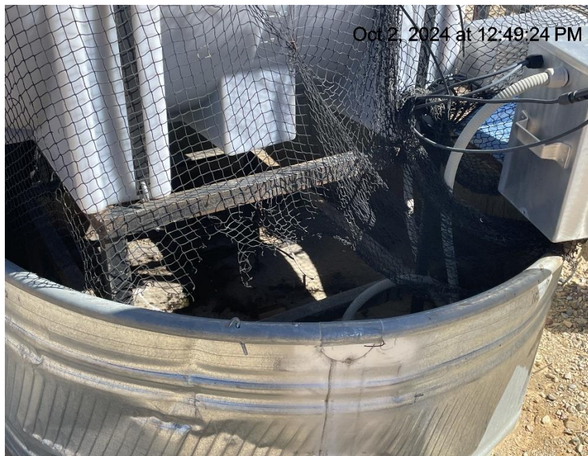
Photo # 3275 Netting/wildlife protection on chemical tank & containment needs maintenance
