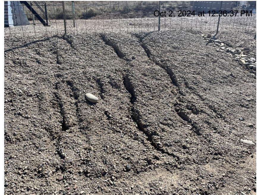
Photo # 3277 Erosion & transport of sediment off location /insufficient BMP's
