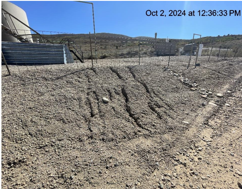
Photo # 3276 Erosion & transport of sediment off location /insufficient BMP's
