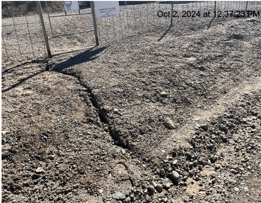
Photo # 3278 Erosion & transport of sediment off location /insufficient BMP's
