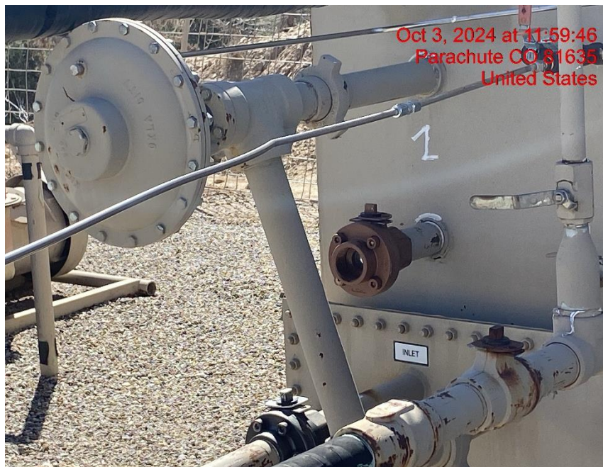
Open-Ended Line on Separator – Photo #03972
