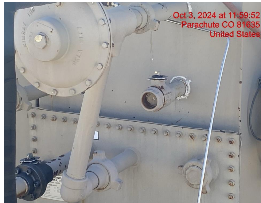
Open-Ended Line on Separator – Photo #03973
