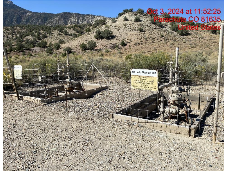
Wellheads/Open Wellhead Cellars – Photo #03962
