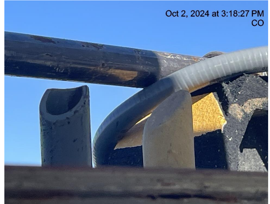
Photo # 3602 PRV vent line does not comply with CECMC pressure safety device rules
