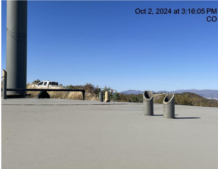
Photo # 3597 PRV & rupture disc vent lines do not comply with CECMC pressure safety device rules
