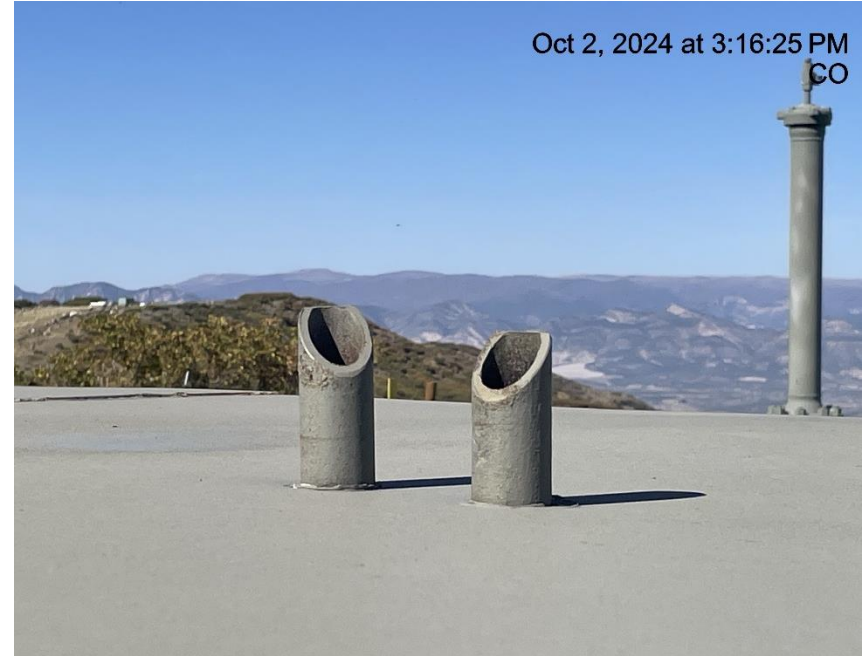
Photo # 3598 PRV & rupture disc vent lines do not comply with CECMC pressure safety device rules
