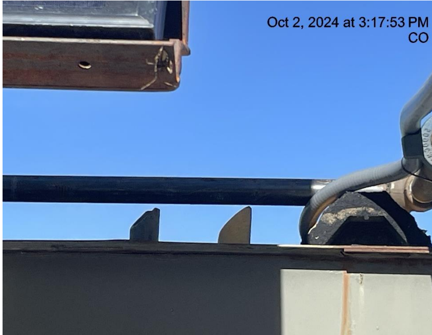
Photo # 3601 PRV vent line does not comply with CECMC pressure safety device rules
