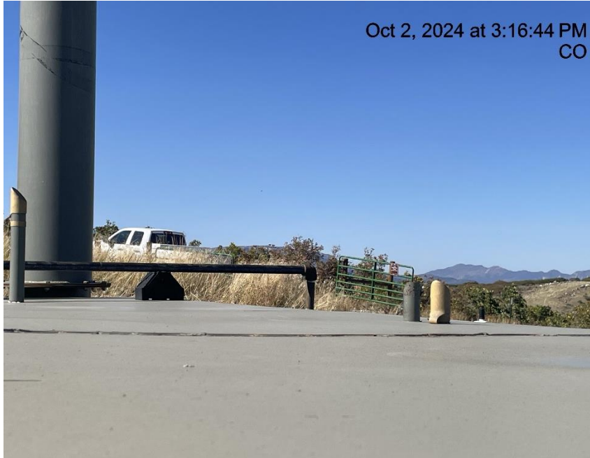
Photo # 3599 PRV vent line does not comply with CECMC pressure safety device rules
