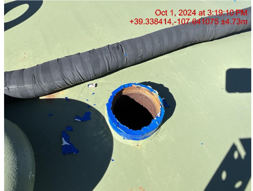
Photo # 6889 Open tank port/wildlife hazard
