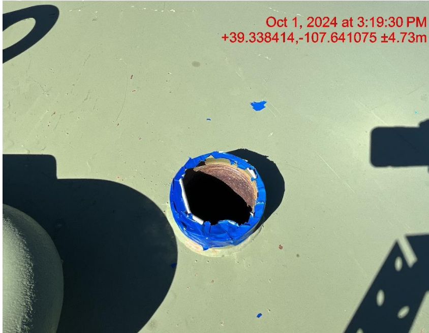
Photo # 6890 Open tank port/wildlife hazard
