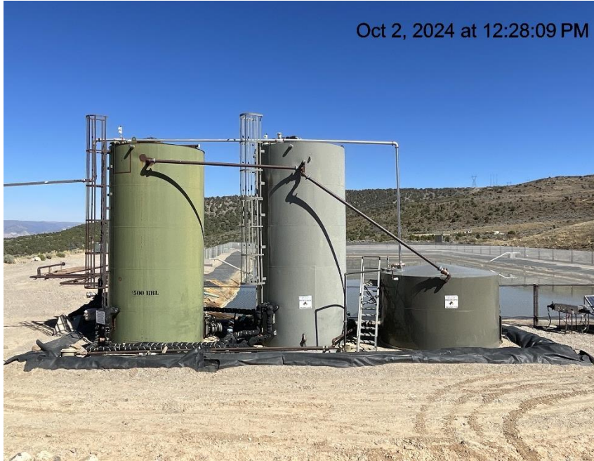
Photo # 3211 Tank battery lacks signage/does not comply with CECMC rules
