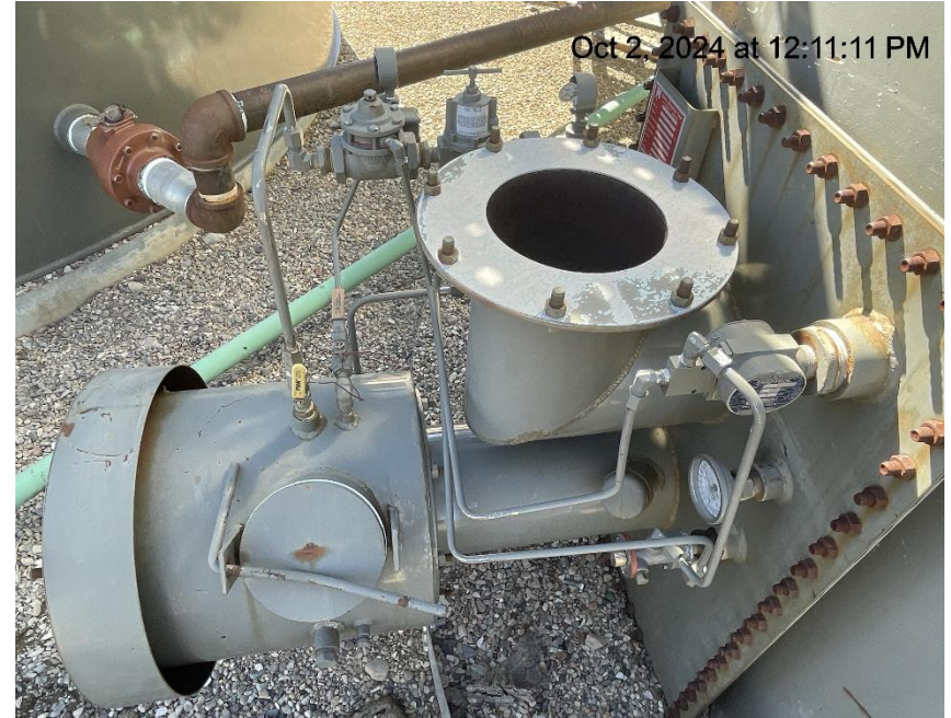
Photo # 3206 Burner exhaust open ended/available for entry by wildlife/wildlife hazard
