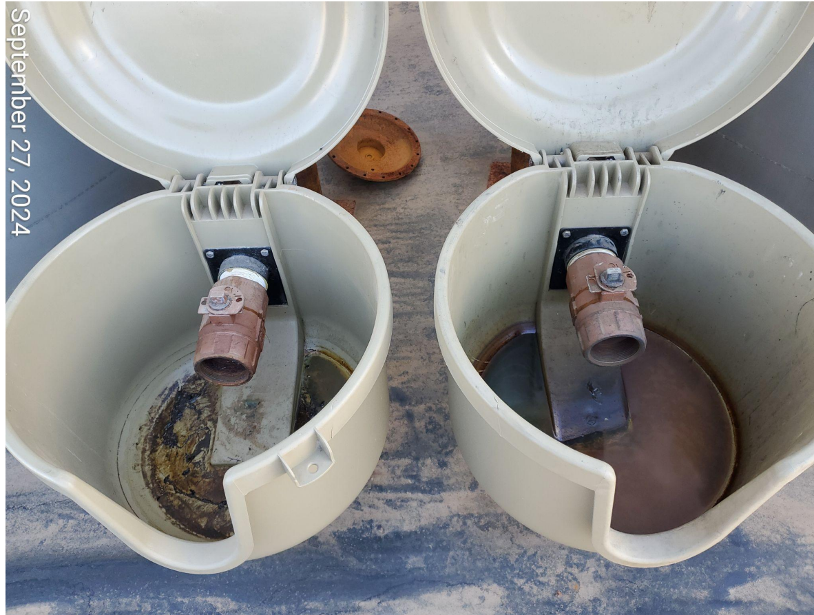
Photo 4: Lines at tanks missing cap/plug.
