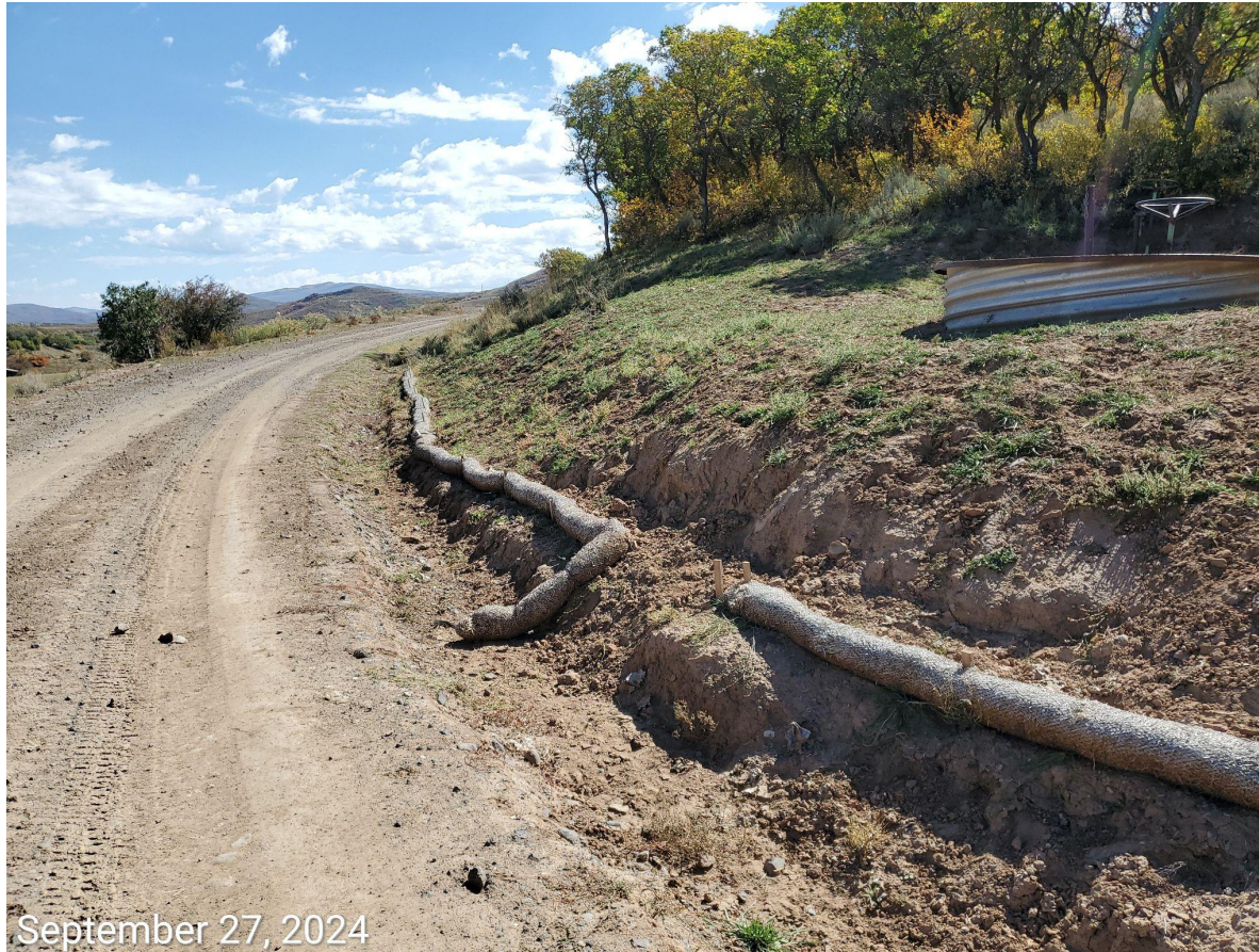
Photo 6: Erosion log in disrepair.
