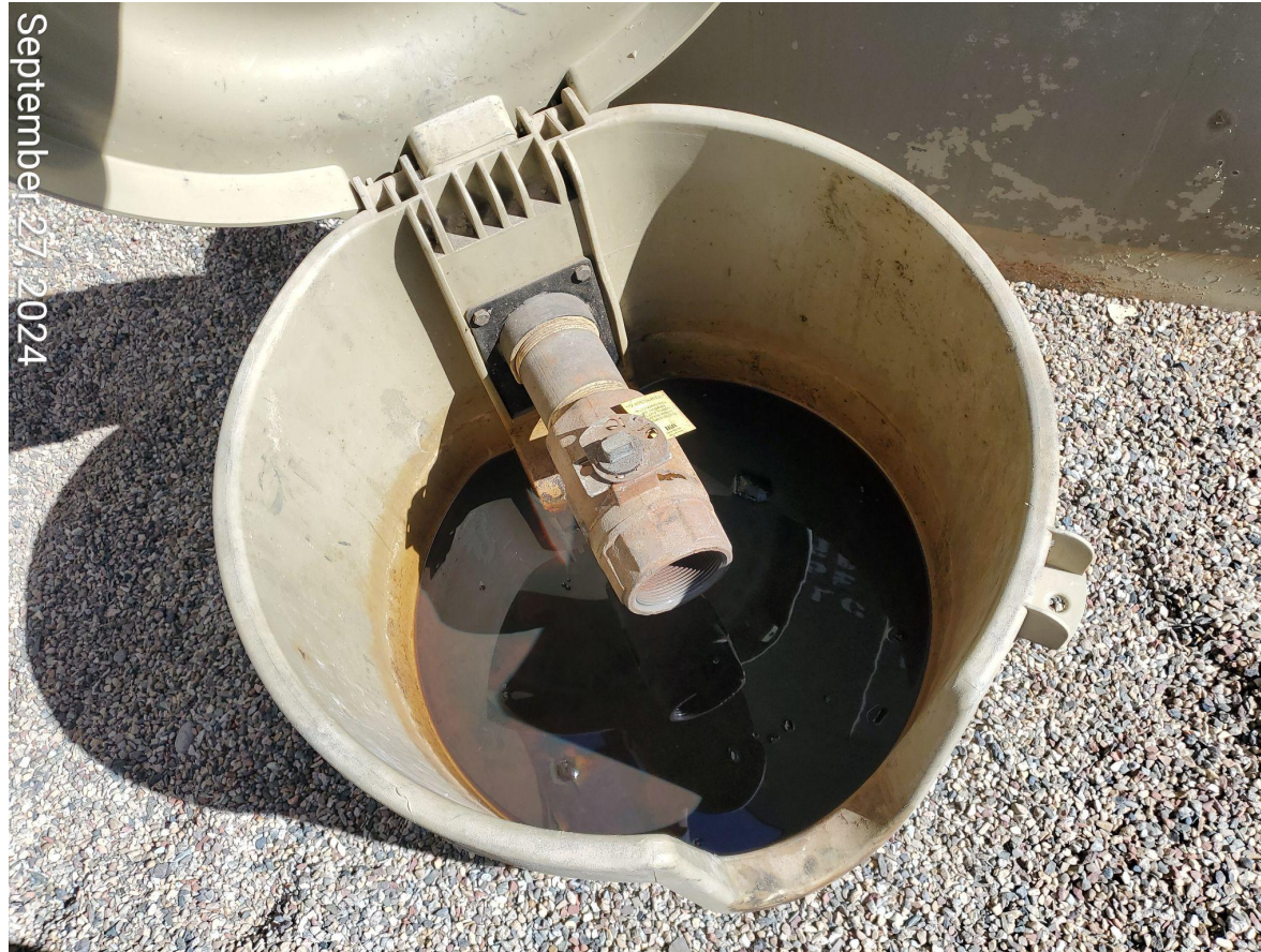
Photo 9: Photo shows line at tank missing cap/plug.
